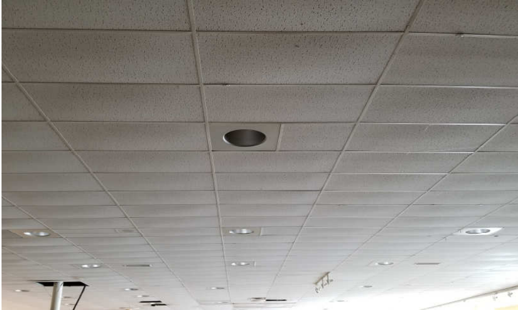
Photo 6: View of acoustic ceiling tiles in the retail floor [i.e. S-3]
