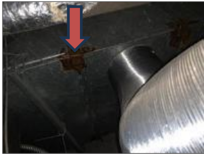
Asbestos-containing reddish brown duct mastic, Room 1172 (Location 5065).
