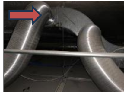
Uninsulated duct, Room 1168 (Location 5063).
