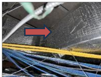
Non-asbestos fibreglass insulated duct jacketed with foil, Saight Atrium Wing Room 2810M and Corridor (Location 204).
