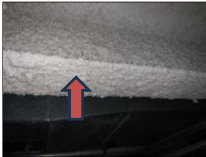
Asbestos-containing light grey/off white fireproofing, Burton Wing Room 2107C (Location 6012).
