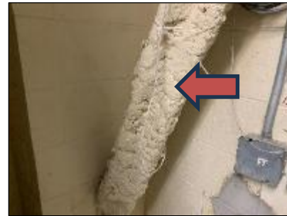
Asbestos-containing white encapsulated fireproofing, Burton Wing Electrical Room 2111 (Location 6058).
