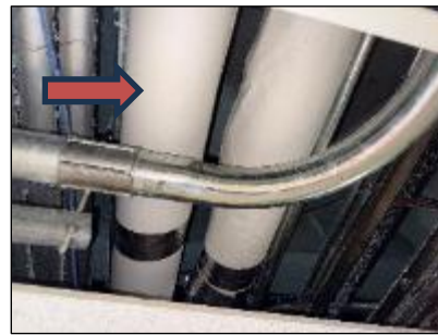
Non-asbestos fiberglass insulated pipes jacketed with paper, Burton Wing 2 nd Floor South Corridor (Location 6004).
