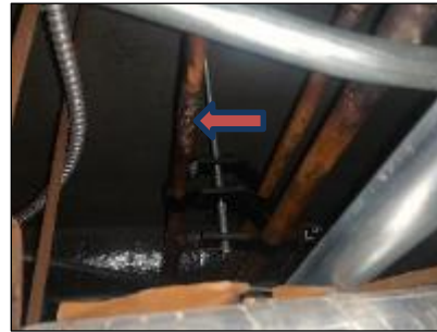
Uninsulated pipes, 2nd Floor Corridor and Elevator Lobby (Location 6001).
