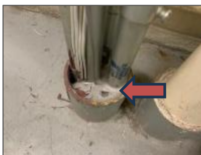
Non-asbestos grey firestop caulking, Electrical Room 2111 (Location 6058).
