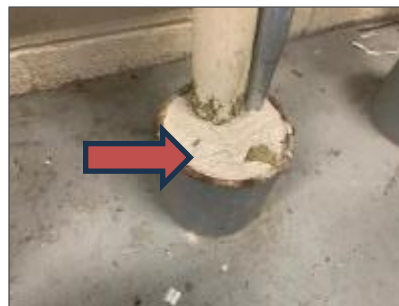
Non-asbestos white firestop caulking, Electrical Room 2111 (Location 6058).
