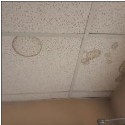
Water staining on non-asbestos ceiling tiles, 2 nd Floor East Corridor (Location 6003).
