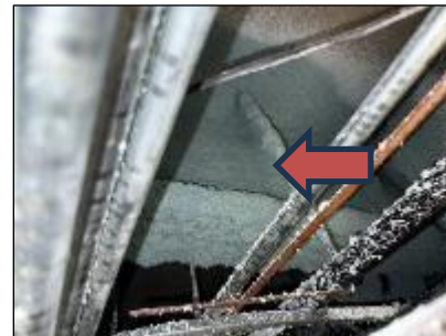
Non-asbestos green fireproofing, Burton Wing 2 nd Floor South Corridor (Location 6004).
