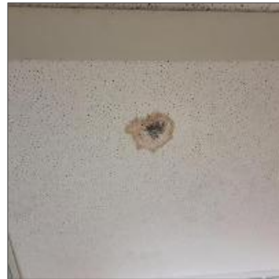
Mould on non-asbestos ceiling tile in the 2 nd Floor South Corridor (Location 6004)
