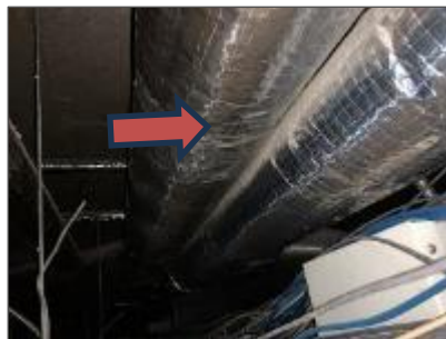
Non-asbestos fibreglass insulated ducts jacketed with foil, 1st Floor South Corridor (Location 5004).
