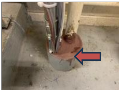
Non-asbestos brownish red firestop caulking, Electrical Room 2111 (Location 6058).
