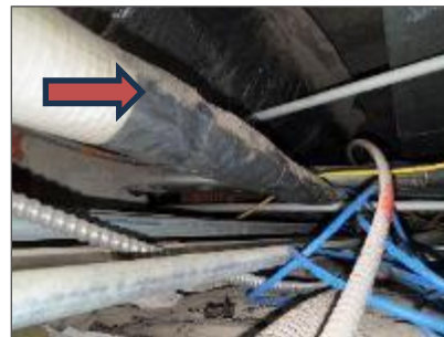
Non-asbestos fibreglass insulated pipe jacketed with foil, Black Wing Corridor S200B (Location 2079).
