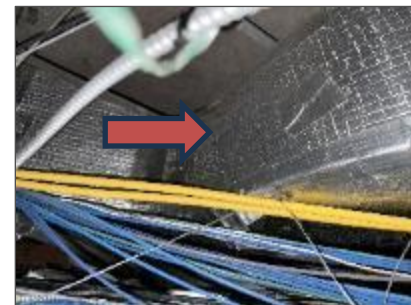
Non-asbestos fibreglass insulated duct jacketed with foil, Black Wing Corridor S200B (Location 2079).
