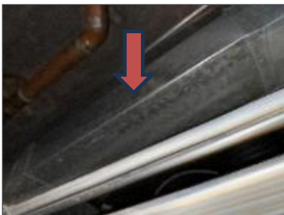
Uninsulated duct, Black Wing Service North Floor Corridor (Location 2035).
