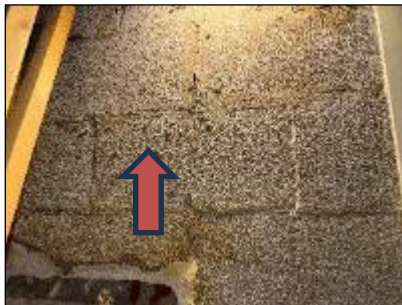
Concrete block wall with asbestos-containing residual fireproofing in pours, Burton Wing Mechanical Shaft/Room S111 (Location 3039).
