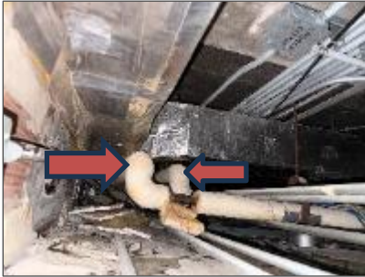
Asbestos-containing paring cement on pipe fittings, Black Wing Service North Floor Corridor (Location 2035).
