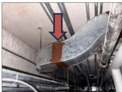
Asbestos-containing reddish brown duct mastic, Saight Atrium Wing Room 2810M and Corridor (Location 204).
