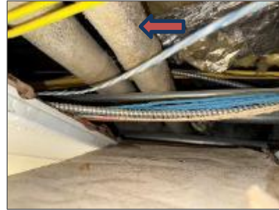
Asbestos-containing aircell pipe insulation, Black Wing Corridor S200B (Location 2079).
