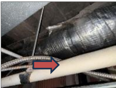
Non-asbestos fibreglass insulated pipes jacketed with paper, Black Wing Corridor S200B (Location 2079).
