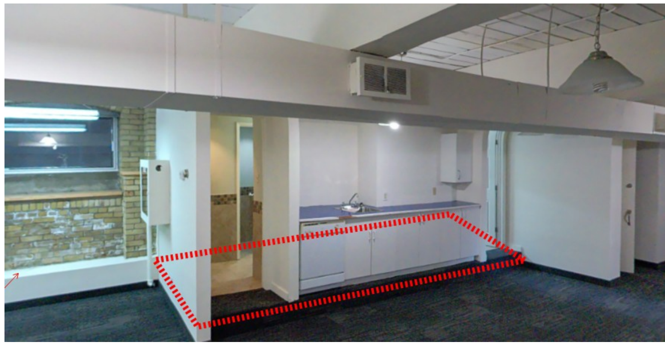
3 PHOTO 1- RAISED FLOOR TO BE REMOVED S2002 Scale: 1 : 25
