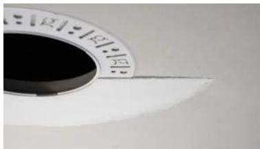
Partially finished mud ring, showing cross-section detail.
