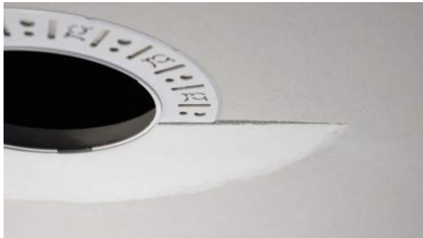
Partially finished mud ring, showing cross-section detail.
