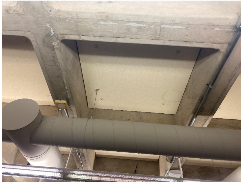
Photo 5 - Presumed asbestos-containing mastic behind roof panels
