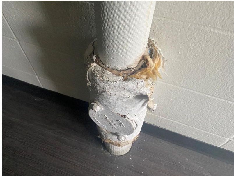
Photo 3 - Presumed asbestos-containing Transite
