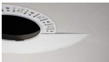
Partially finished mud ring, showing cross-section detail.
