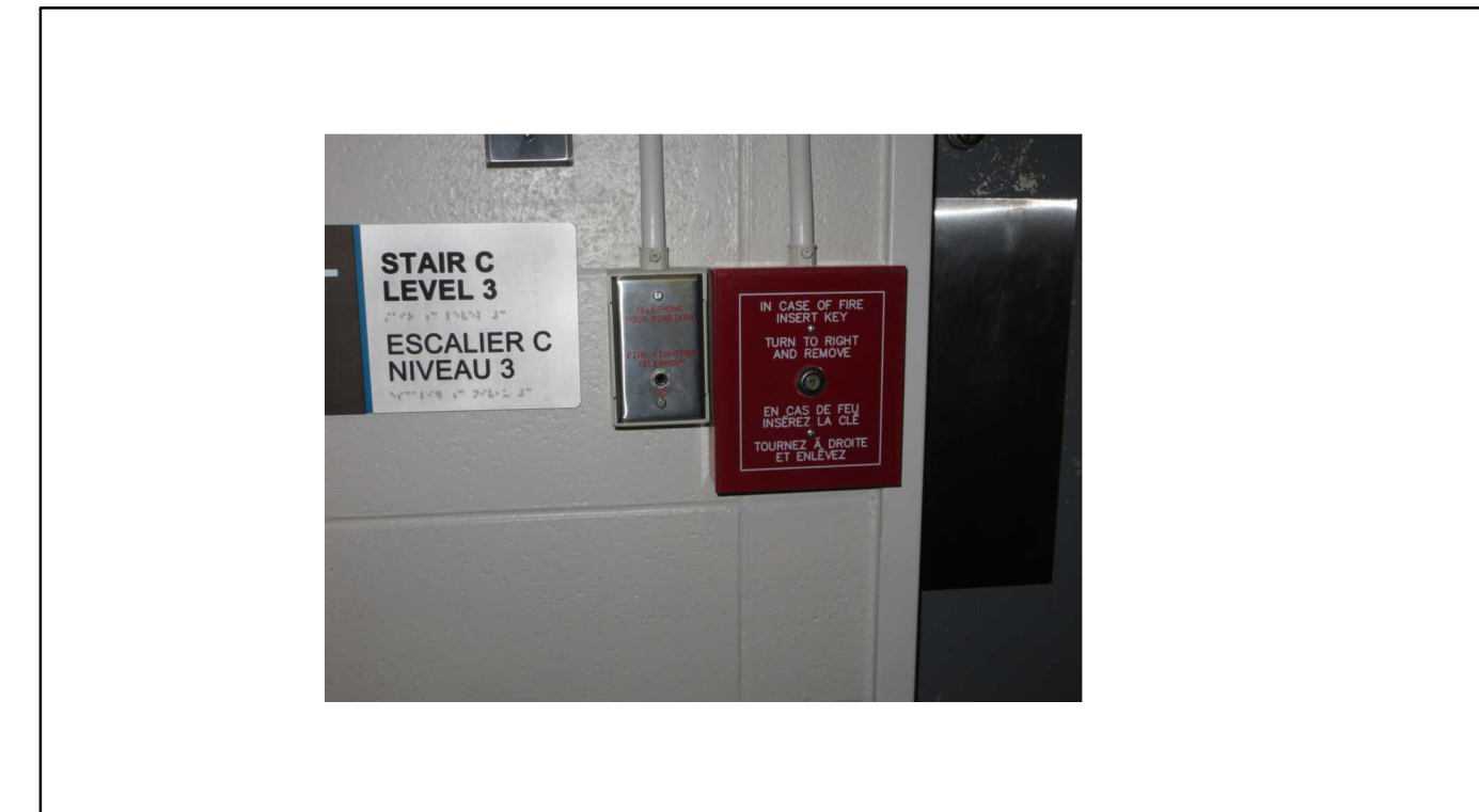
7 PHOTO OF EXISTING KEY SWITCH/MAN PULL STATION SCALE: N.T.S.
