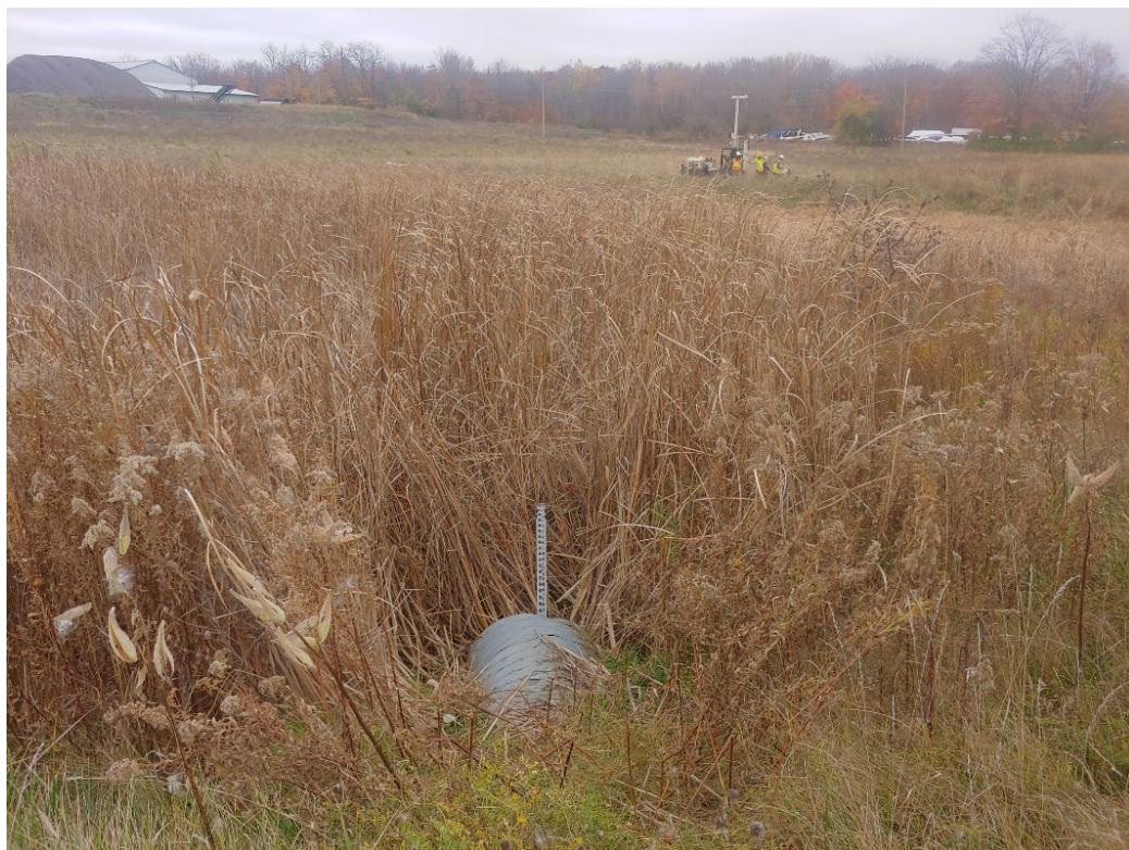
Picture 12: Culvert to Discharge Water into The Municipal Line.
