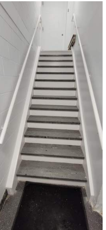
PHOTO 21: STAIR C, INSTALL NEW TEXTURAL WARNING STRIPS AND TACTILE ATTENTION INDICATORS
