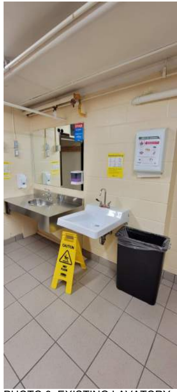
PHOTO 8: EXISTING LAVATORY TO REMAIN INSULATE EXISTING PIPES AT WOMEN'S CHANGEROOM 122
