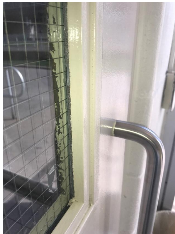
Photos 1, 2 – View of non-asbestos containing black putty inside the door.
