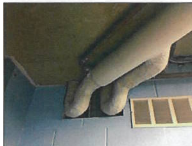
Photo #2: Typical non-asbestos fibreglass pipe insulation with canvas jacketing on the sanitary system found throughout the lower level of the building.
