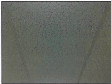
Photo #4: Non-asbestos acoustic ceiling tile 1, 24"x48" with flecks and pinholes, (Samples A0003A-C)
