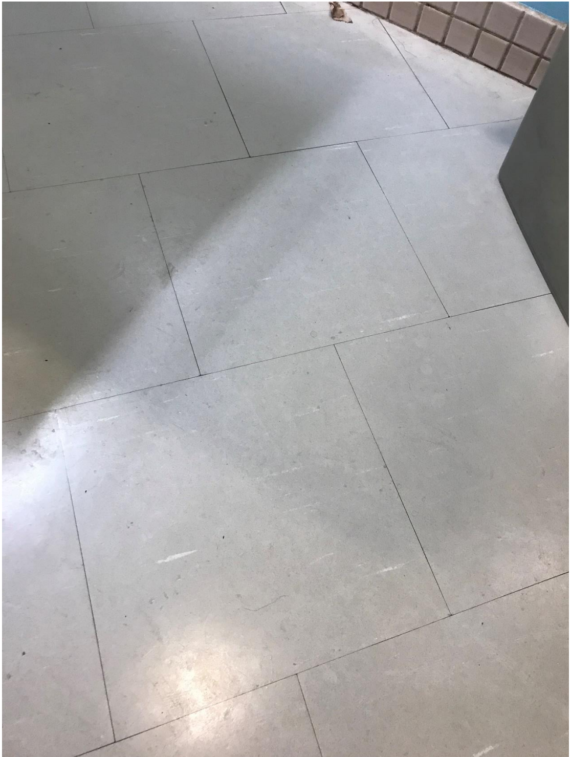
Photo 1 – View of the asbestos-containing Vinyl Floor Tile 1 (12"x12" Grey with White Lines) observed in the washroom on first floor.
