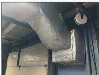
Photo #3: Duct in garage with non-asbestos fibreglass insulation with foil jacketing.
