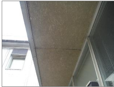
Photo 2: Assumed asbestos-containing Transite board on exterior soffits.
