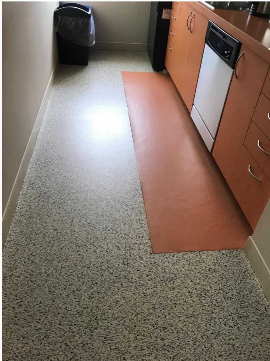
Photo 2 – View of non-asbestos containing Vinyl Sheet Flooring 1, and Vinyl Sheet Flooring 5 observed at the Site.
