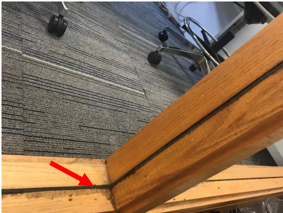
Photos 1, 2 – View of the asbestos-containing grey putty between wall frame and glass observed in the Meeting Room on main floor.
