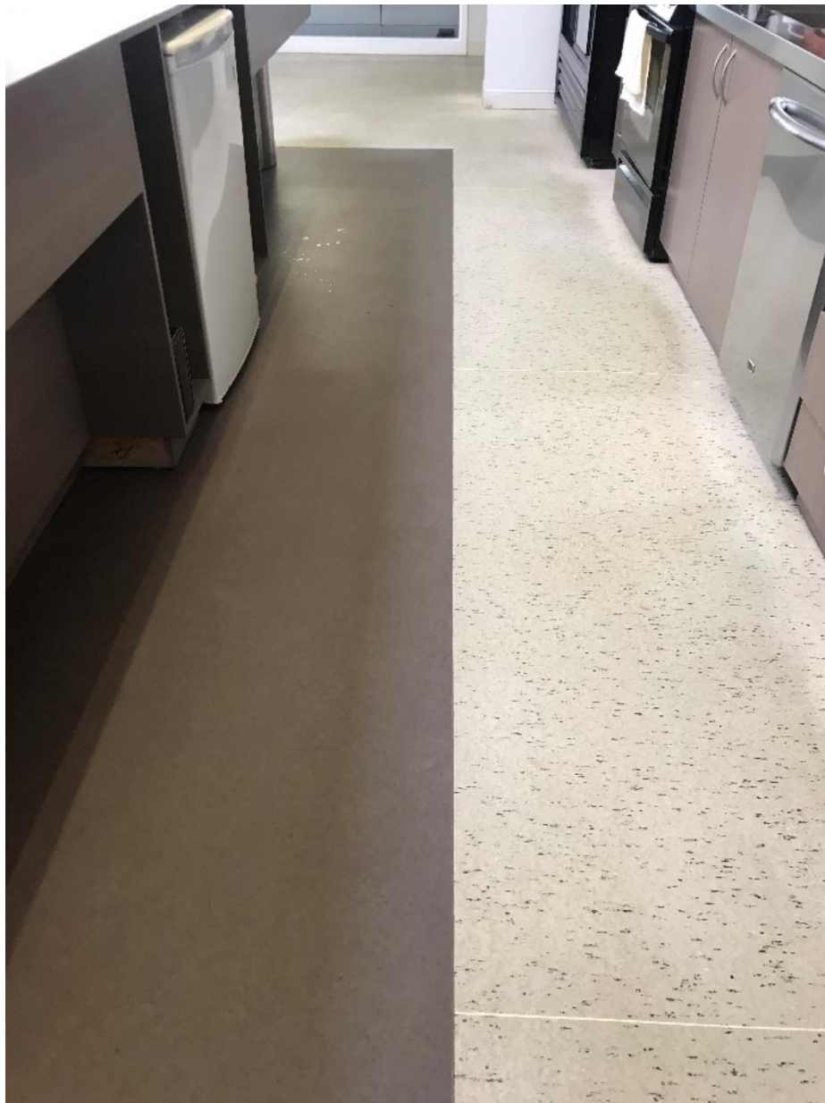
Photo 1 – View of non-asbestos containing Vinyl Sheet Flooring 2 and Vinyl Sheet Flooring 7 observed at the Site.
