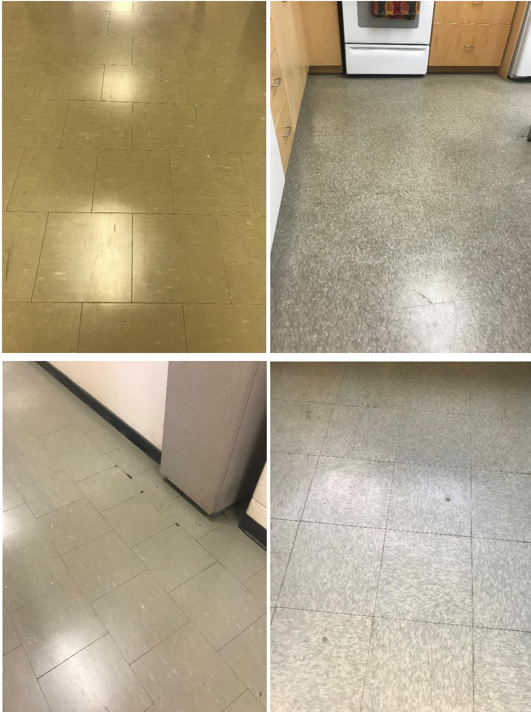
Photos 1 to 4 – Examples of the various non-asbestos containing vinyl floor tiles observed in the building.
