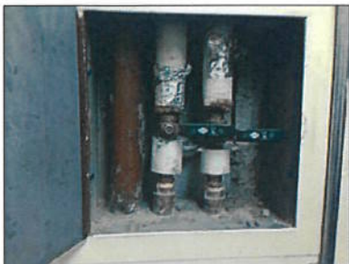
Photo #1: Typical non-asbestos fibreglass pipe insulation with canvas jacketing on the domestic hot and cold water systems found throughout the building.
