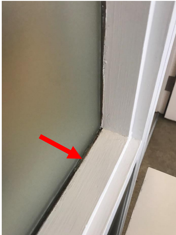
Photos 3, 4 - View of the asbestos-containing grey putty between wall frame and door observed in the Kitchenette on 2 nd floor.
