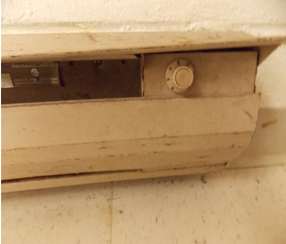
D3050 Heat Transfer Terminal and Packaged Units:- Close-up of aged baseboard heater
