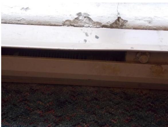
Impact damage on baseboard heater in the open space of the Library
