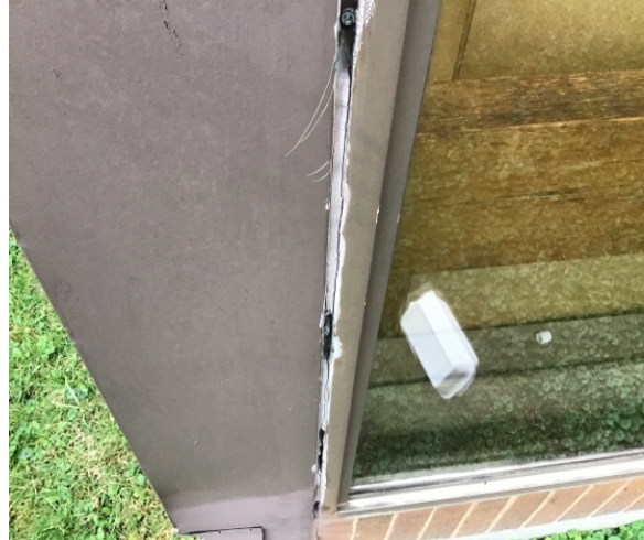
B2011.1 Exterior Wall Sealant:- View of Exterior Sealant
