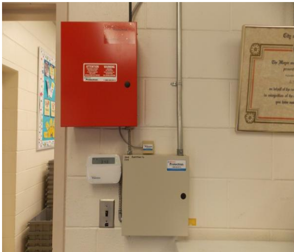
D5030 Communications and Security Systems:- Security system control panel in the Staff Room
