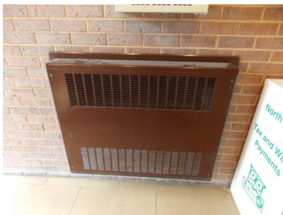
Forced flow heater in the main entrance vestibule
