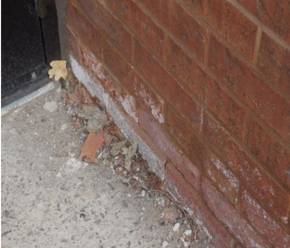
B2011 Exterior Wall Construction:- Close-up of spalling brick and efflorescence
