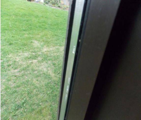
B2021 Windows:- Close-up of typical window metal spacer and glazing seal
