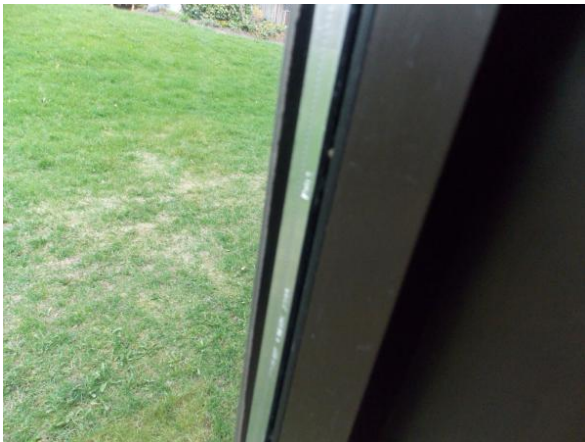
Close-up of typical window metal spacer and glazing seal
