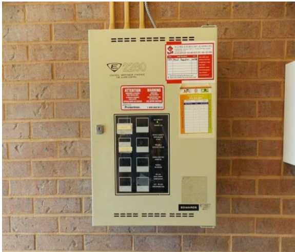
D5030 Communications and Security Systems:- General view of fire alarm control panel
