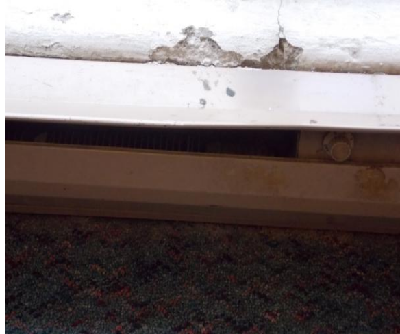
D3050 Heat Transfer Terminal and Packaged Units:- Impact damage on baseboard heater in the open space of the Library
