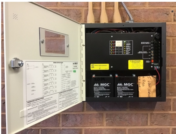
General view of fire alarm control panel
