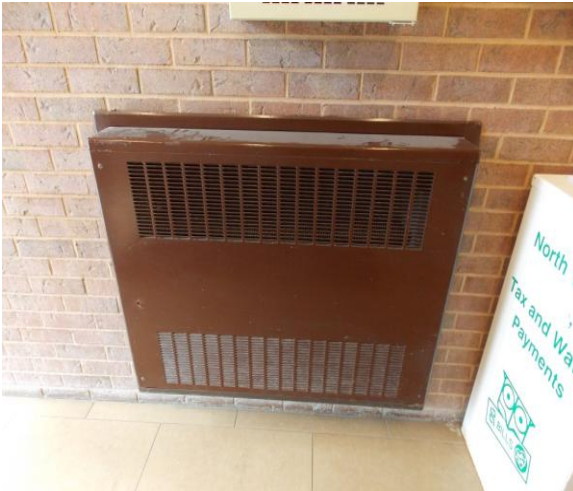
D3050 Heat Transfer Terminal and Packaged Units:- Forced flow heater in the main entrance vestibule
