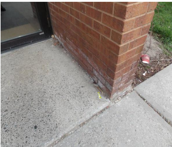
B2011 Exterior Wall Construction:- Efflorescence near the main entrance
