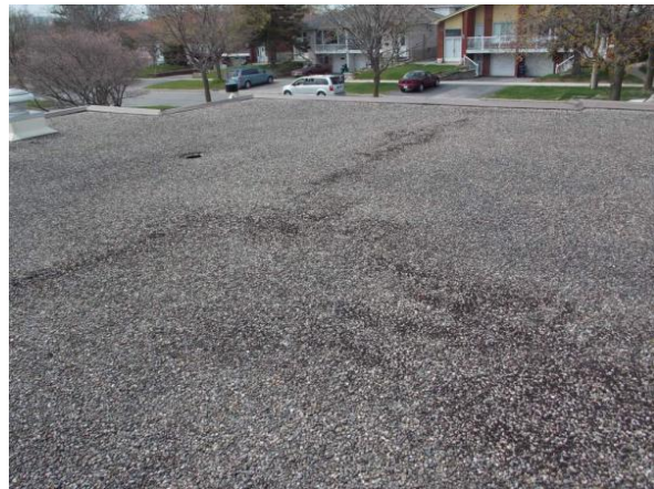
Some asphalt migration on the roof
