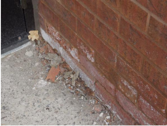
Close-up of spalling brick and efflorescence
