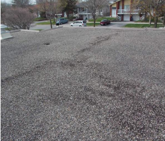
B3011 Roof Finishes:- Some asphalt migration on the roof
