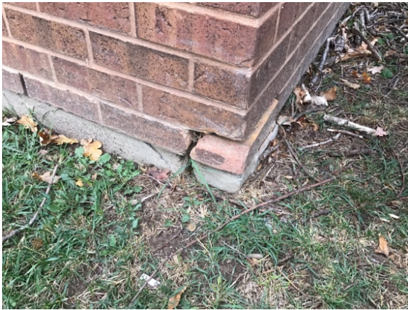
Close-up of spalling brick and efflorescence
