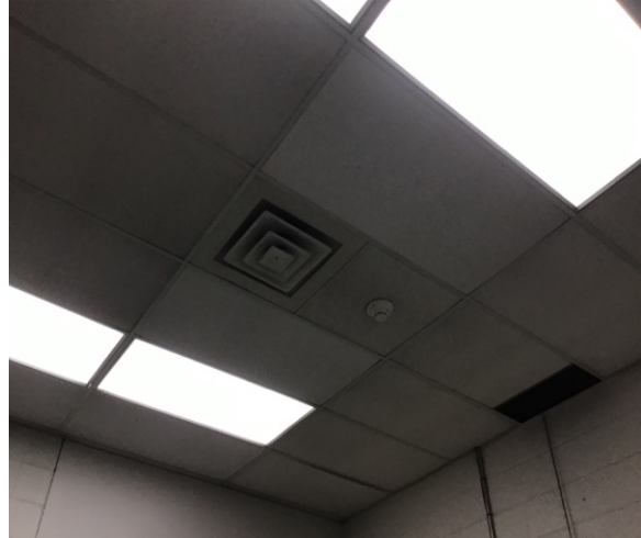
C3031 Ceiling Finishes:- View of Suspended Acoustic Panels
