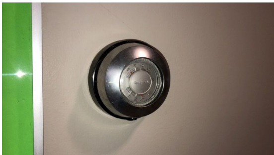
Photo 2: Thermostat with mercury bulb.
