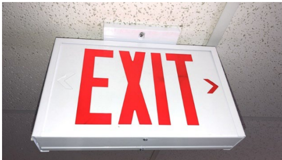
Photo 1: Emergency lighting with suspect lead-acid batteries.
