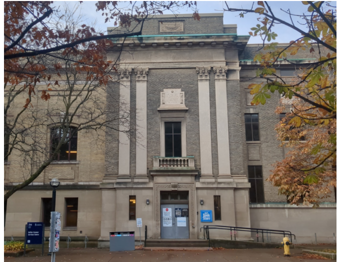
Figure 28: St. George Entrance (November 2024, EVOQ). Existing wood doors have already been removed to shop for rehabilitation to accommodate the interior demolition already underway in the first stage of work.
