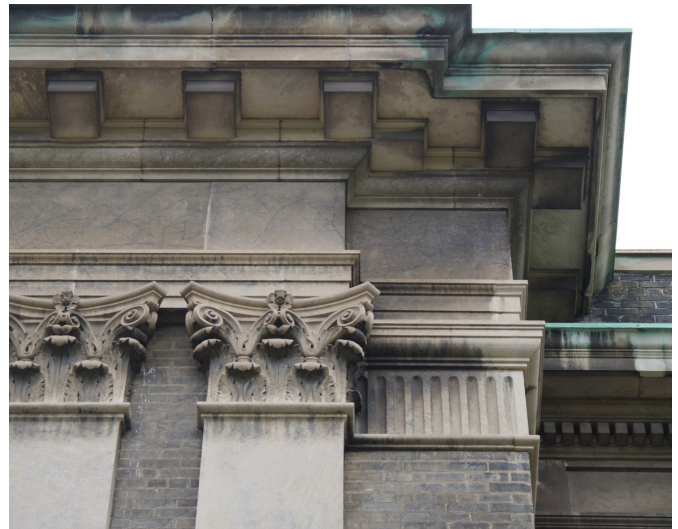
Figure 19: Cupric (copper) staining and atmospheric soiling (2020, EVOQ)
