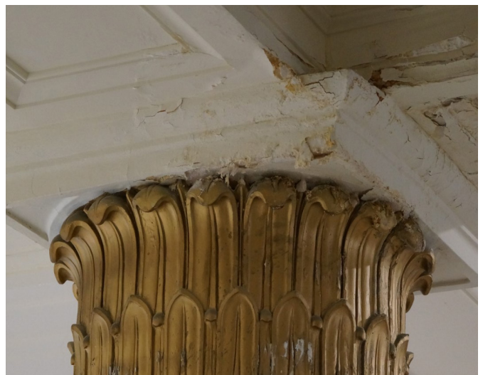
Figure 24: Plaster deterioration on ceilings and columns (2020, EVOQ)
