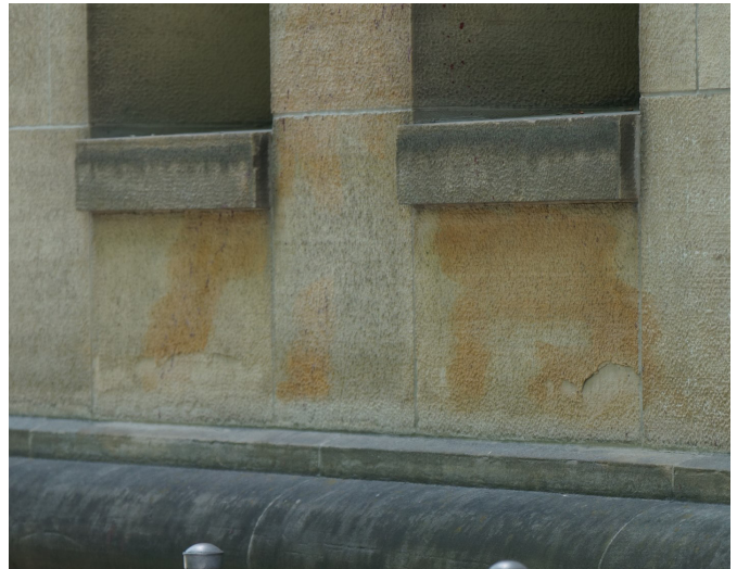
Figure 20: Atmospheric soiling and scaling of stonework (2020, EVOQ)
