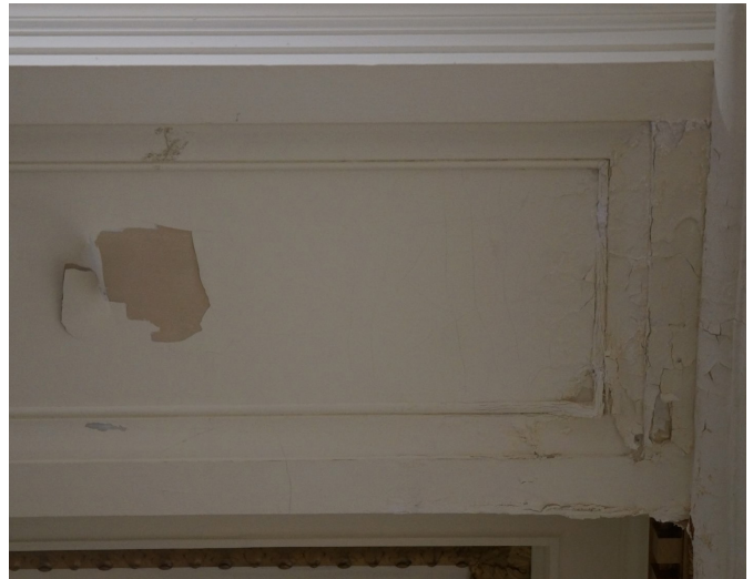
Figure 23: Plaster delamination and water damage (2020, EVOQ)
