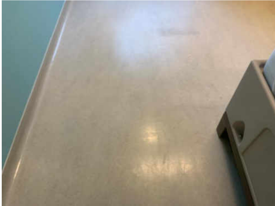
V0016 Floor, Mastic underneath vinyl sheet flooring, Room 7A29 (Location #: 710)
