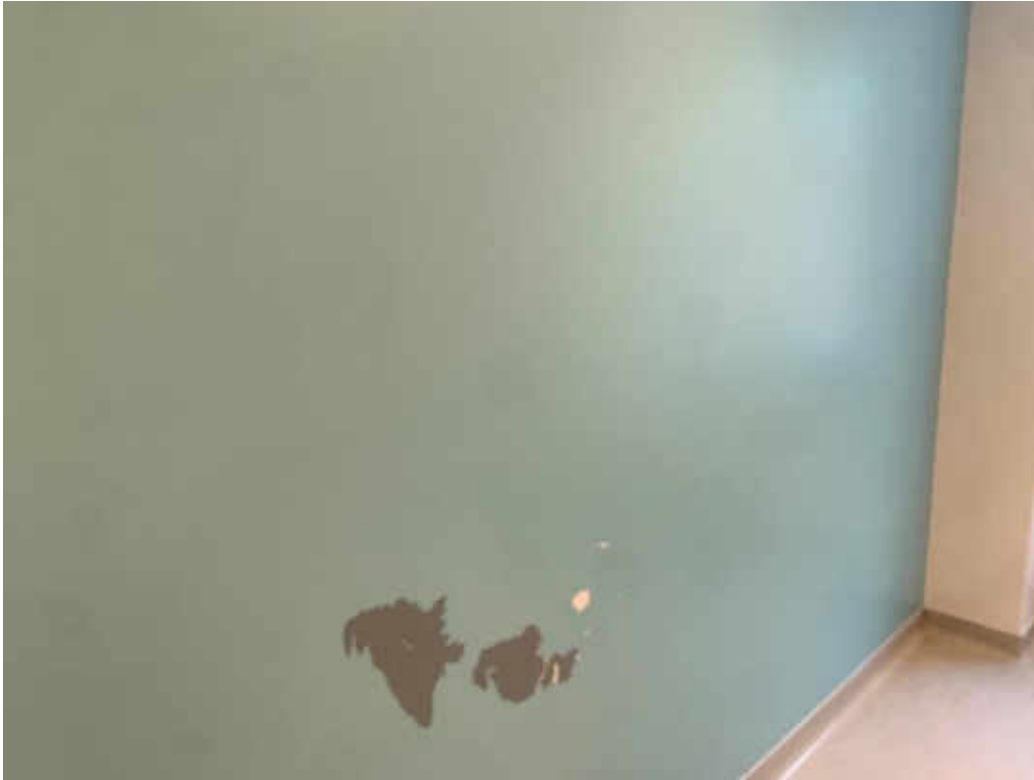
V0022, (Lead, None), Light blue paint on drywall wall, Room 7A29 (Location #: 710)
