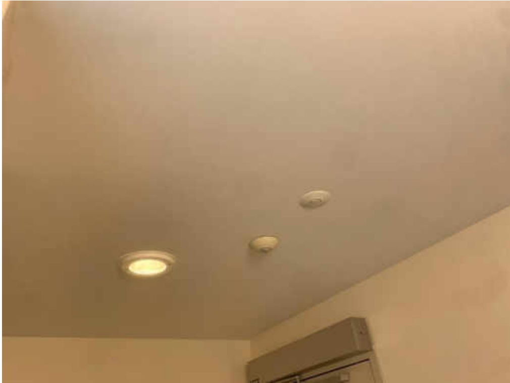
V0000, (None) Ceiling, Drywall joint compound on drywall ceiling, Washroom (Location #: 712)
