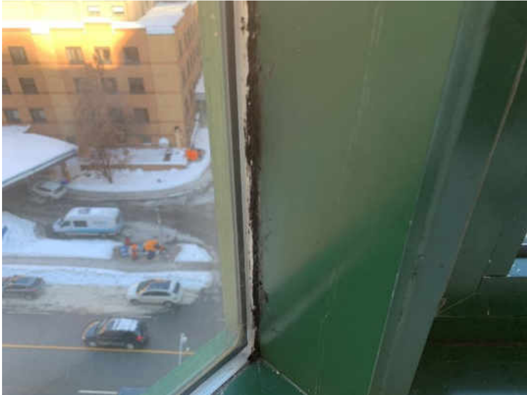
V0029, Other, Black butyl caulking, Corridor and Reception Area (Location #: 709)
