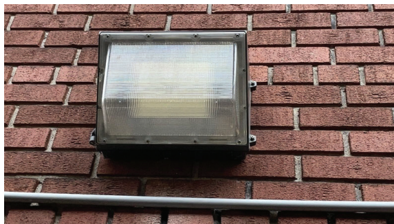
Photo 11: Example of high intensity discharge light fixture suspected to contain PCB ballast.
