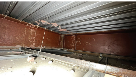
Photo 5: Example of structural steel primer suspected to contain lead.
