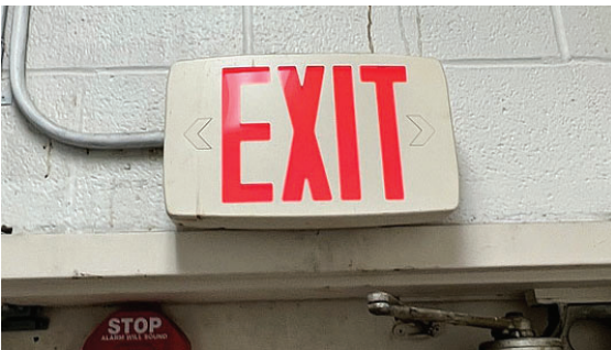
Photo 3: Example of emergency exit sign and lighting suspected to contain lead-acid batteries.
