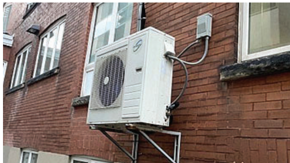
Photo 13: Example of air conditioning unit suspected to contain ODS.
