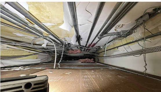
Photo 1: Example of loose and flaking paint.
