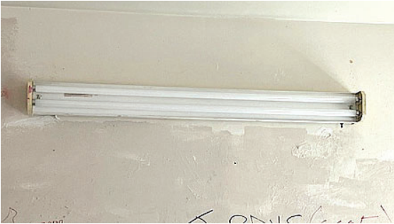
Photo 8: Example of light fixture with fluorescent light tubes suspected to contain mercury (vapour form).
