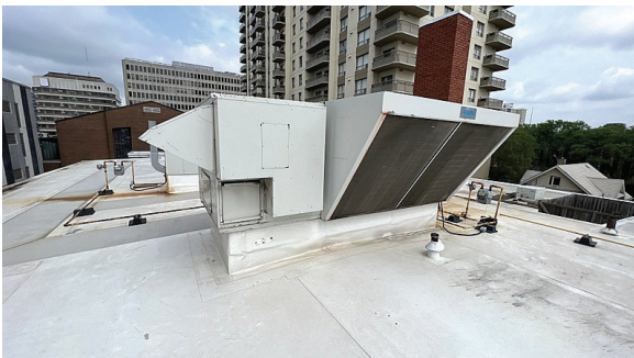
Photo 12: Example of rooftop HVAC units suspected to contain ODS.
