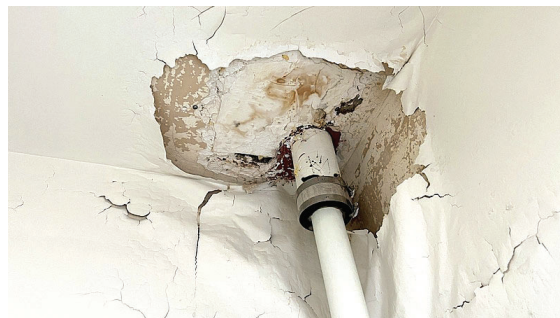
Photo 2: Example of loose and flaking paint.
