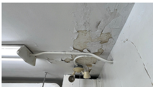
Photo 16: Example of water damage to paint coating on ceiling in Room 332 (L3-23).
