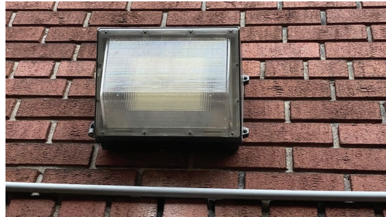
Photo 9: Example of high intensity discharge light fixture suspected to contain mercury (vapour form).
