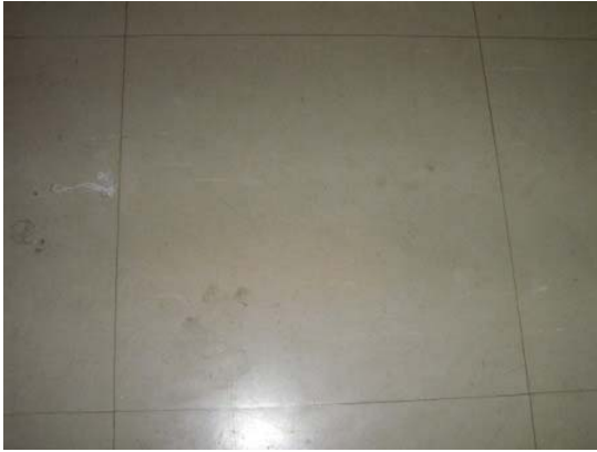
Vinyl floor tile, 12"x12", beige, pattern of white streaks, location NG29, Clean Linen, contains no asbestos (sample 003A-C)
