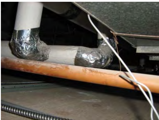
Photo 5 – Fibreglass insulated pipe with paper covering and foil taped elbows
