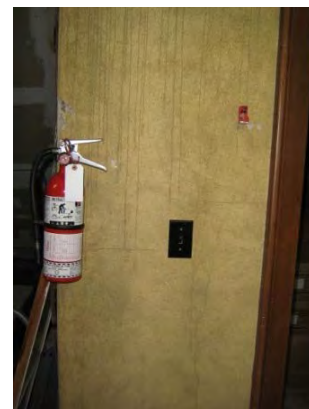
Plaster, containing asbestos, painted yellow, (sample 011A), attic level of Residence building
