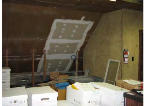
Typical view of new drywall in Residence Attic level, drywall compound contains no asbestos due to date of installation
