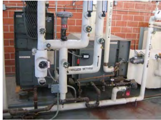
Photo 8 – Pipes insulated with fibreglass insulation
