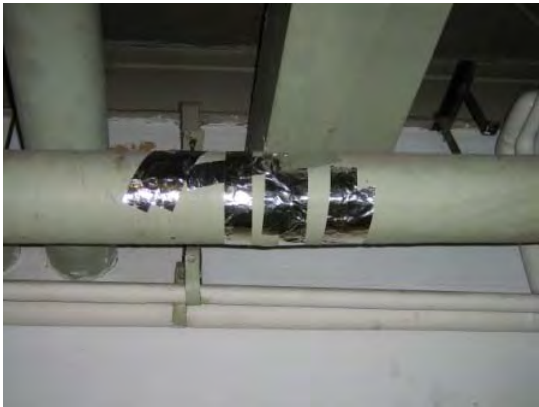
Sweatwrap not containing asbestos (samples 001A-C), parging cement on seams containing asbestos (sample 002A), room NG20
