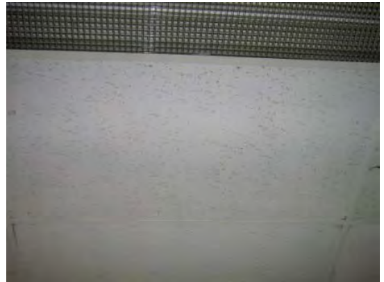
Acoustic ceiling tile, 2'x4', white with pattern of medium fissures and pinholes, contains asbestos (sample 008A), location – blue storage shed
