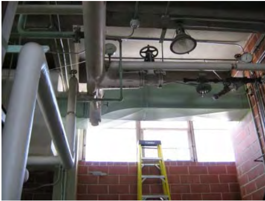
Photo 7 – Pipes insulated with fibreglass insulation
