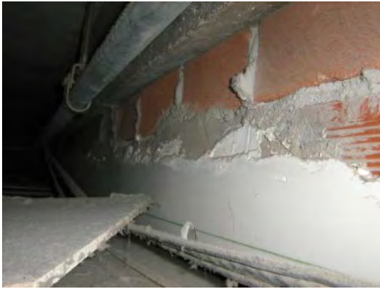
Photo 1 – Plaster on brick – Sample S002
