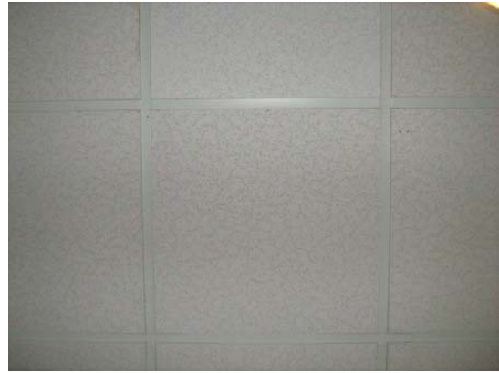
Photo 2 – 2' x 2' Acoustic ceiling tile – Sample S001
