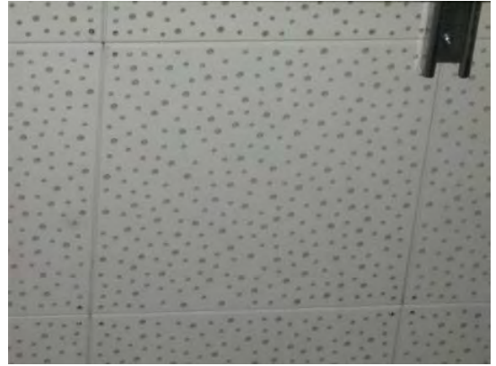
Screwed-on acoustic ceiling tile, 1'x1', white, pattern of large and medium round holes, location NG02, Bell Telecom room, contains no asbestos (sample 005A-C)
