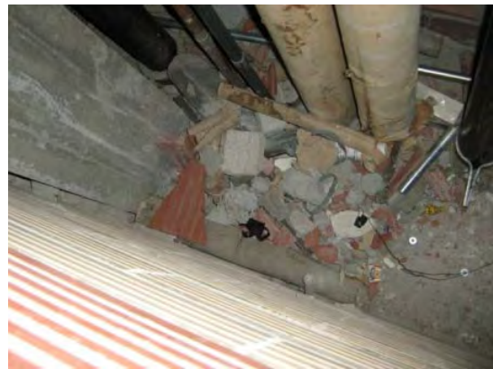
Photo 10 – Debris inside pipe chase
