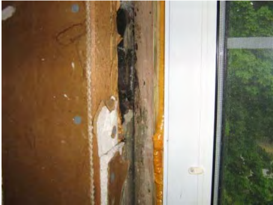
Black caulking, around window, location: Attic level of Residence building, contains no asbestos (sample 010A-C)
