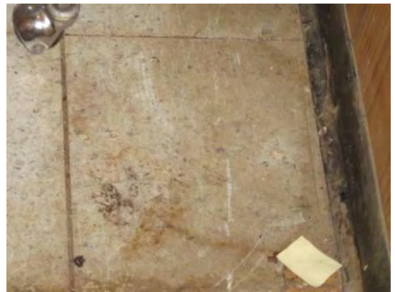
Vinyl floor tile, 12"x12", gray with black flecks, present in old bathroom area in Blue Shed, assumed to contain asbestos
