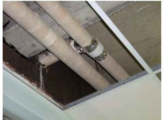
Typical above-ceiling view in South Wing. Note fiberglass straight sections with canvas covering, fiberglass fittings with paper and foil tape coverings, location: corridor outside room S110
