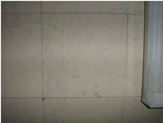
Glued-on acoustic ceiling tile, 1'x1', white, pattern of widthwise fissures, location SG38, Library, contains no asbestos (sample 007A-C)
