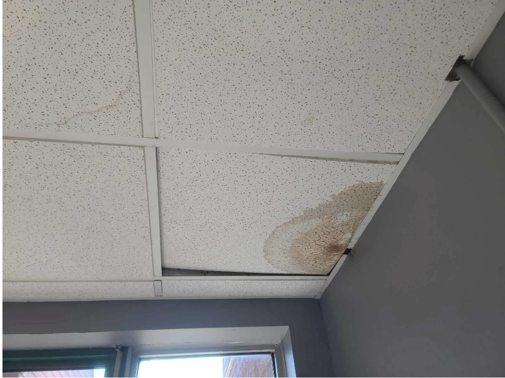
Photo 7: Mould Impacted ceiling tiles in Location 1-045.
