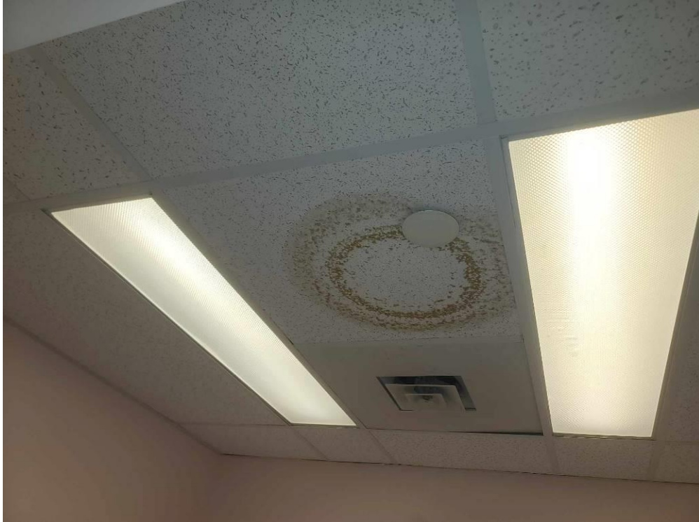
Photo 13: Mould Impacted ceiling tiles in Location 2-066.
