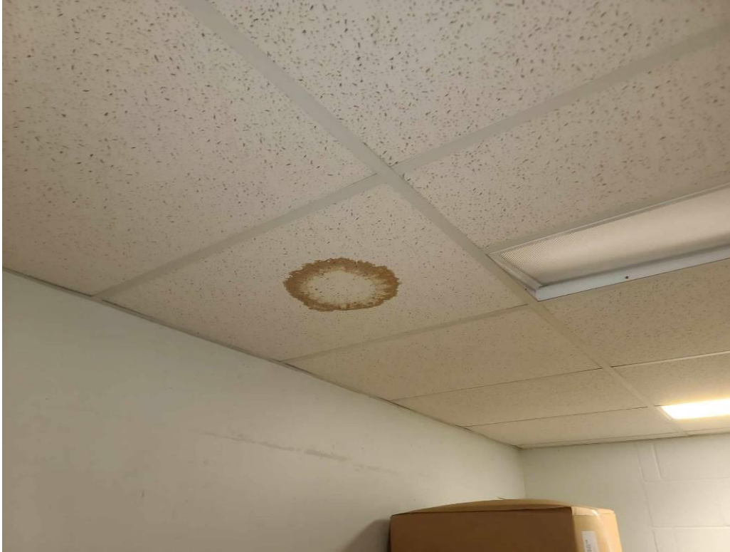
Photo 3: Mould Impacted ceiling tiles in Location B-007.
