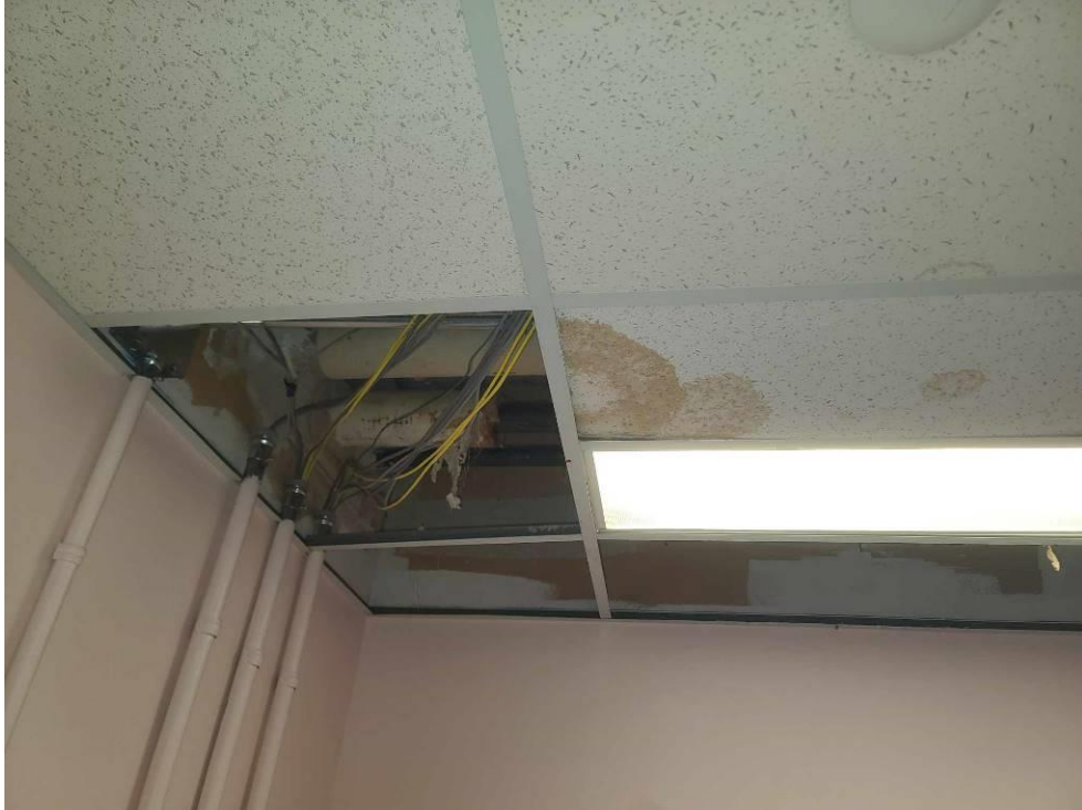
Photo 9: Mould Impacted ceiling tiles in Location 3-026.
