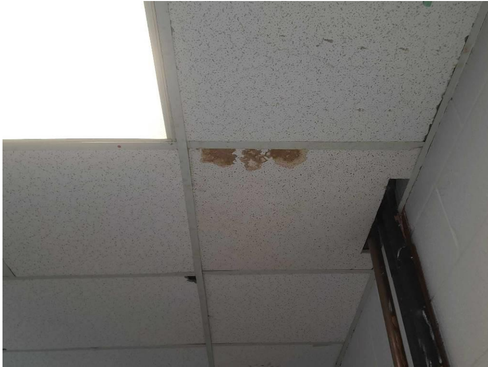
Photo 11: Mould Impacted ceiling tiles in Location 1-039.
