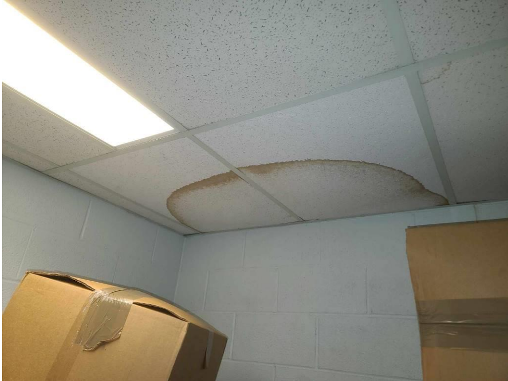
Photo 5: Mould Impacted ceiling tiles in Location B-007.
