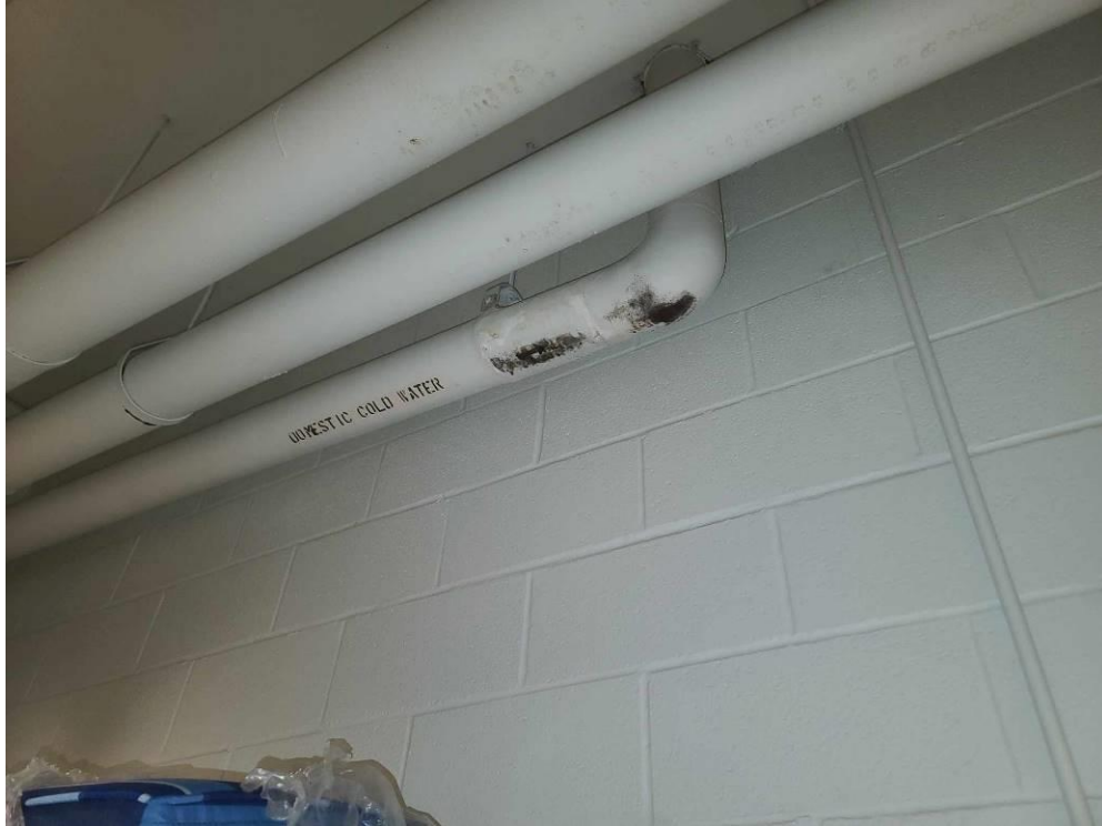
Photo 1: Mould Impacted pipe insulation in Location B-009.
