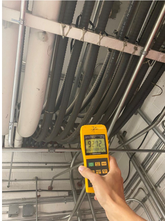
Figure 9: A.C. Magnetic field readings taken below single conductor cables located in main electrical room.
