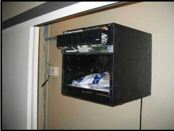
Currently the HDSL was not moved over from other location. This is the High Park supervisor's house. Issue here, rack was larger than expected by the client, so it should have been placed in the basement out of the way. That is why the closet now has doors. Rack is 11U Rack. There is about 12 connections in Total.
