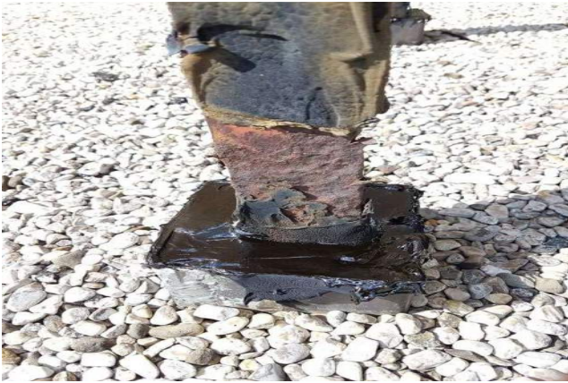
Topped up pitch pans with fresh mastic
