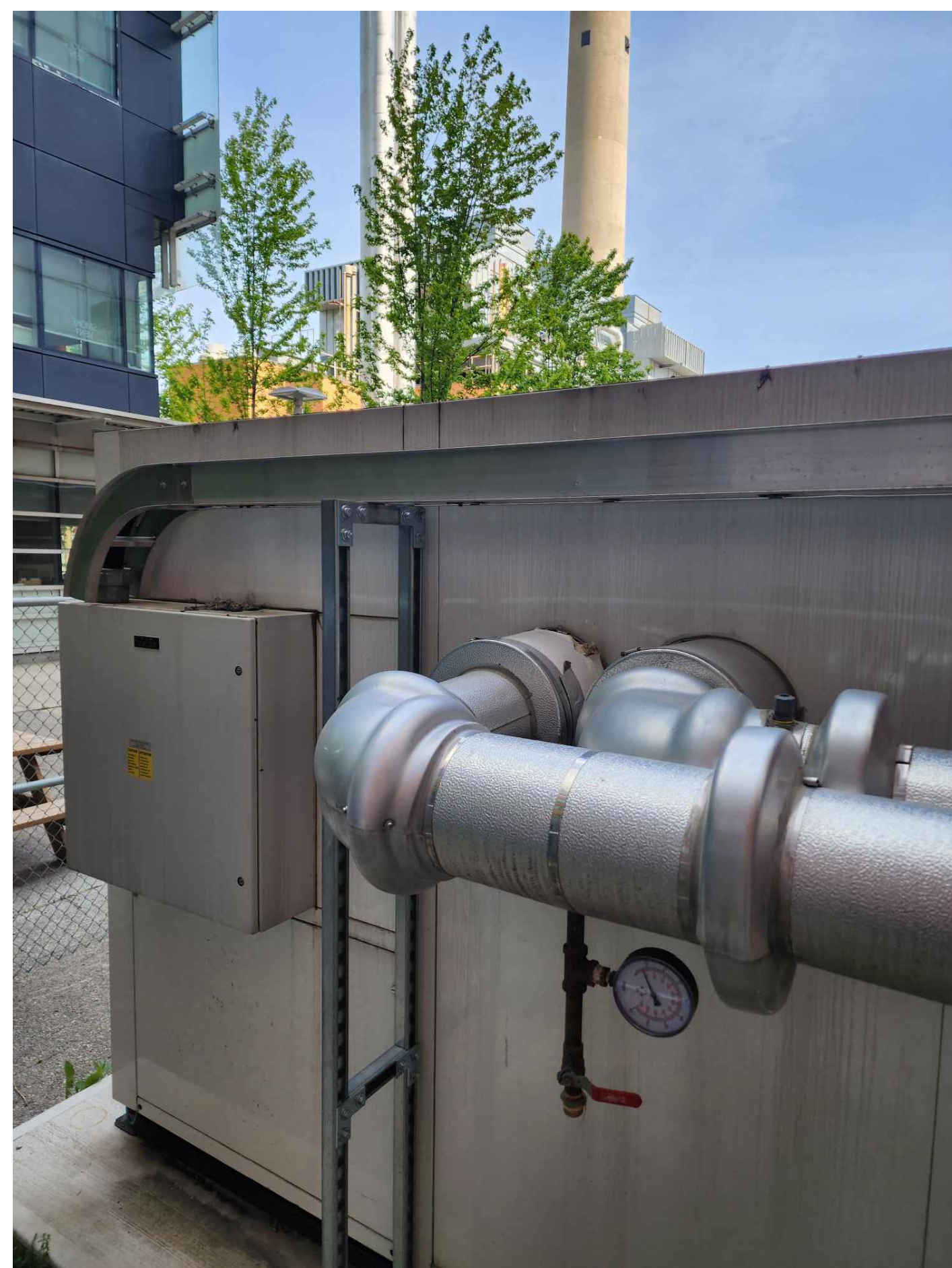
EXISTING CHILLER TEMPERATURE GAUGE
