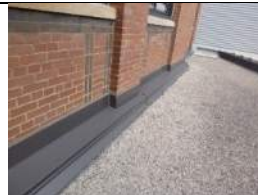
View of counter flashing at wall
