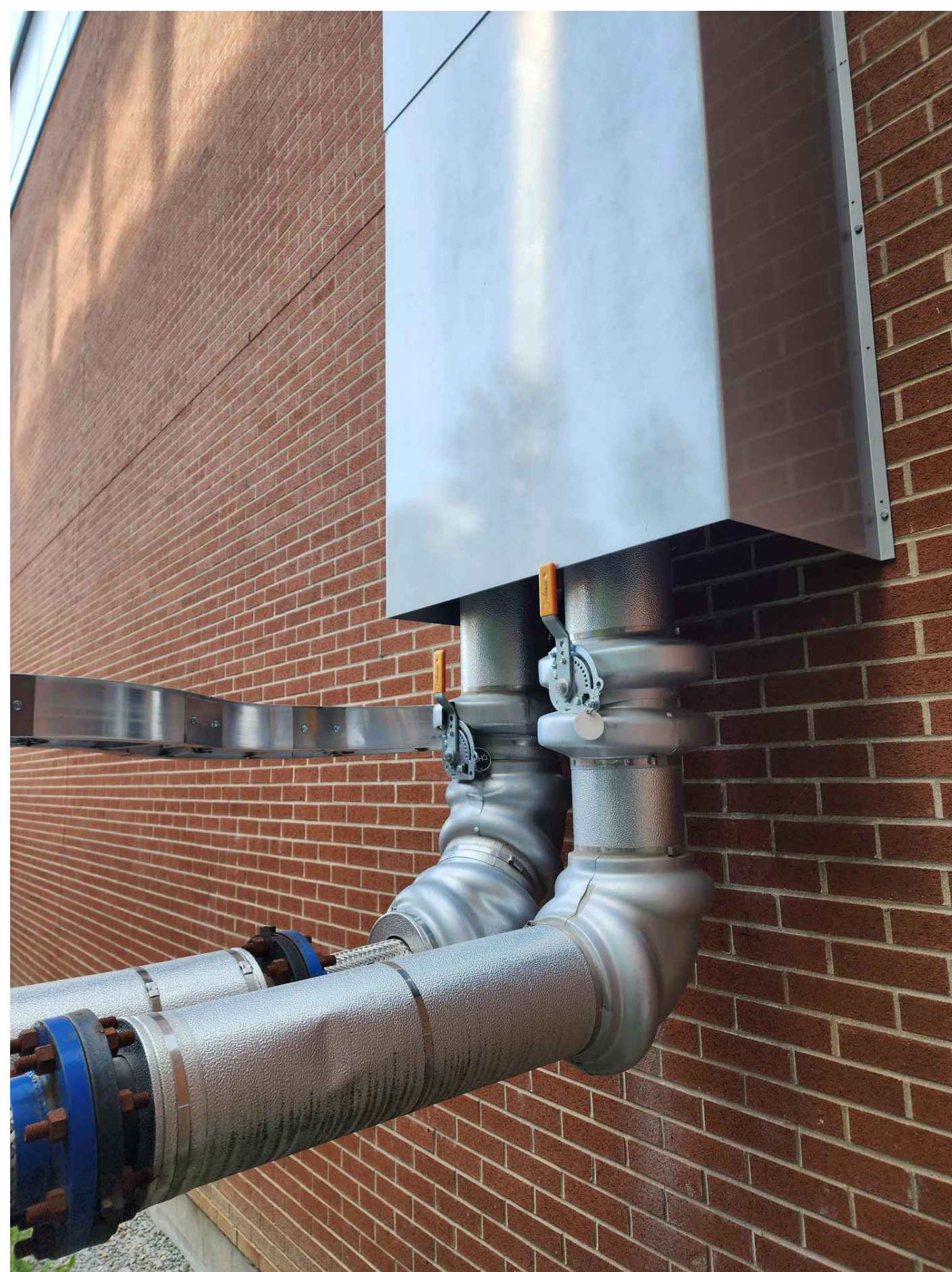
EXISTING CHILLER ISOLATION VALVES
