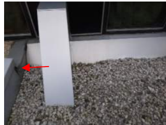
Flashing joint open
