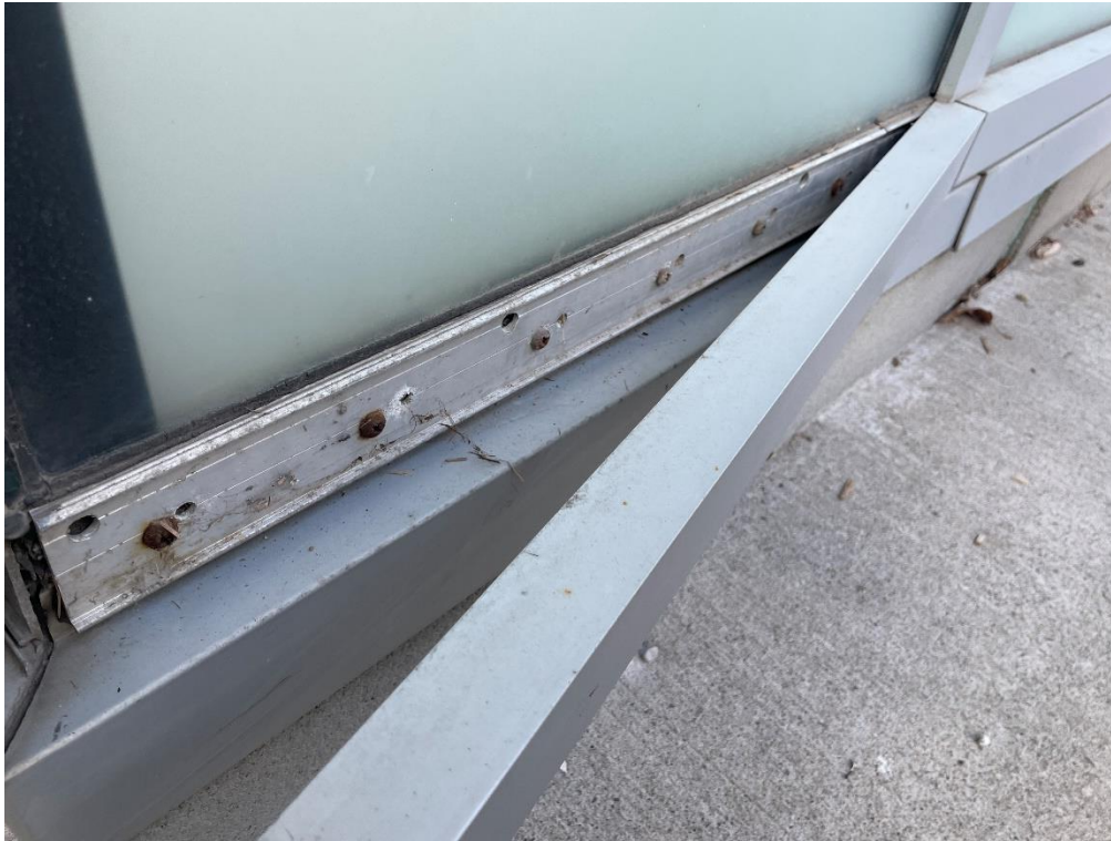
Photograph No. 15 Corroded fasteners at pressure plates, and inadequate weep holes.
