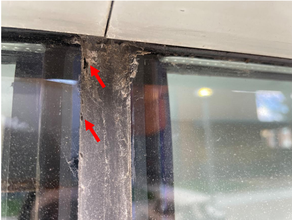
Photograph No. 11 Discontinuous sealant
