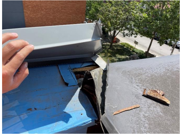
Image 24 – Poor membrane tie-in
