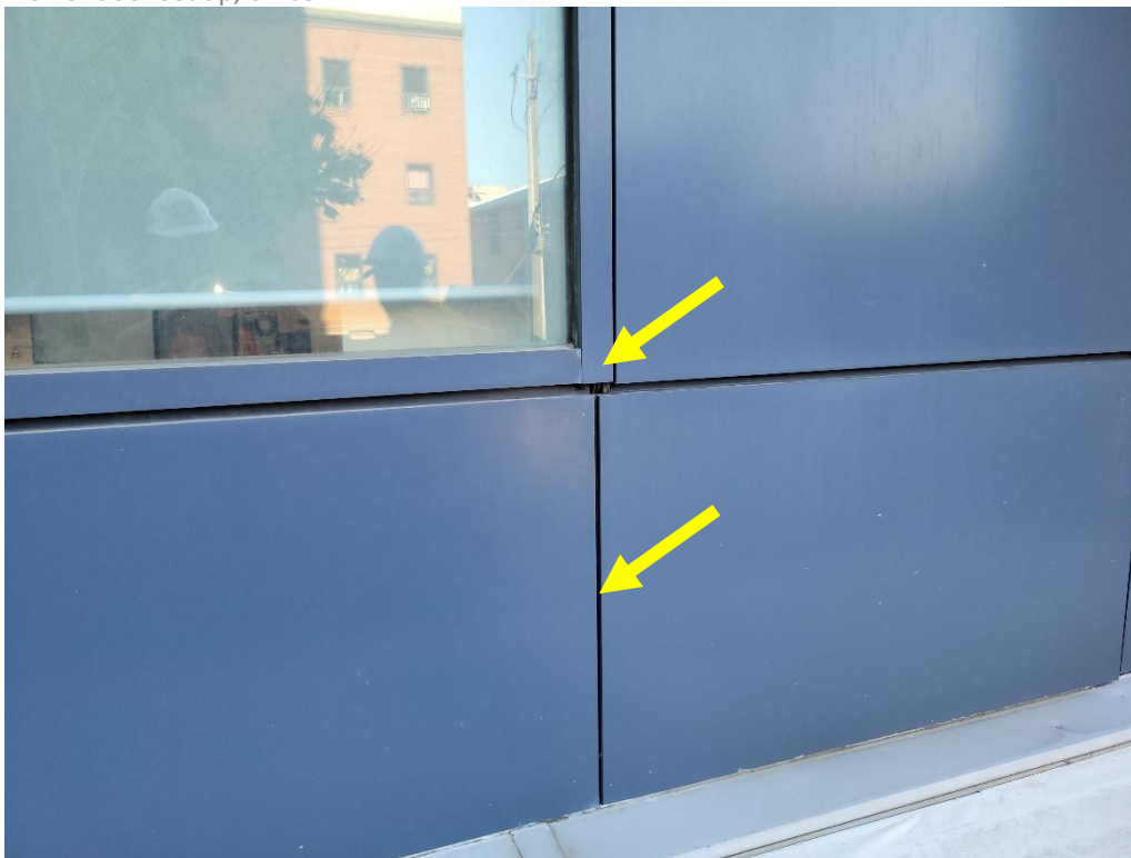
Photograph No. 42 Water penetration occurring above canopy, at arrow locations.
