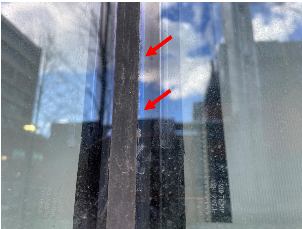
Photograph No. 12 Exposed spacer bar.
