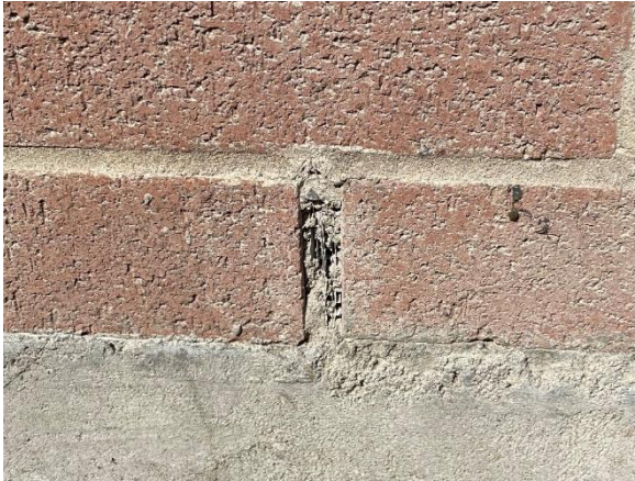
Image 9 – Weep holes obstructed
