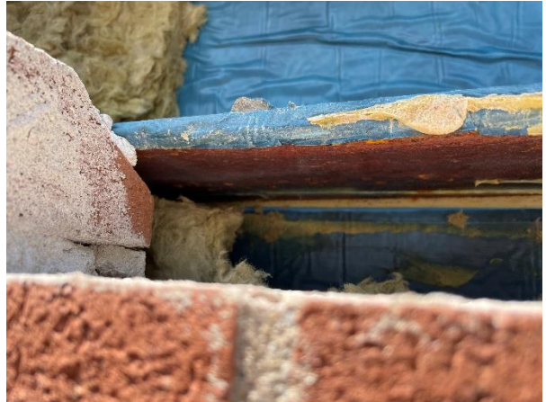
Image 18 – Masonry cut to accommodate angle
