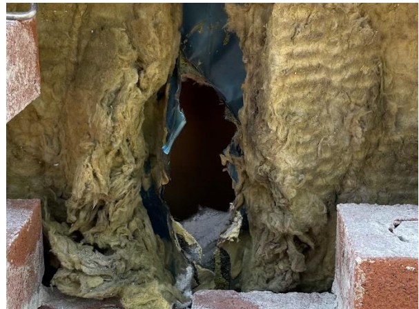
Image 20 – Hole through exterior sheathing
