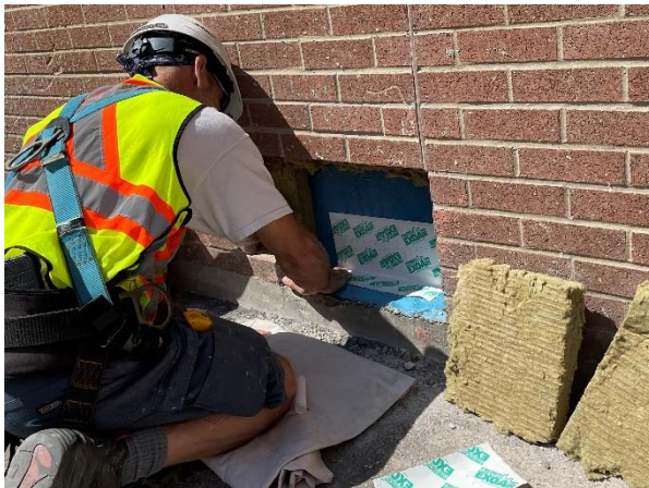
Image 27 – Example membrane patch applied
