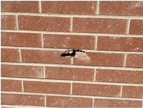
Image 5 – Damaged brick units
