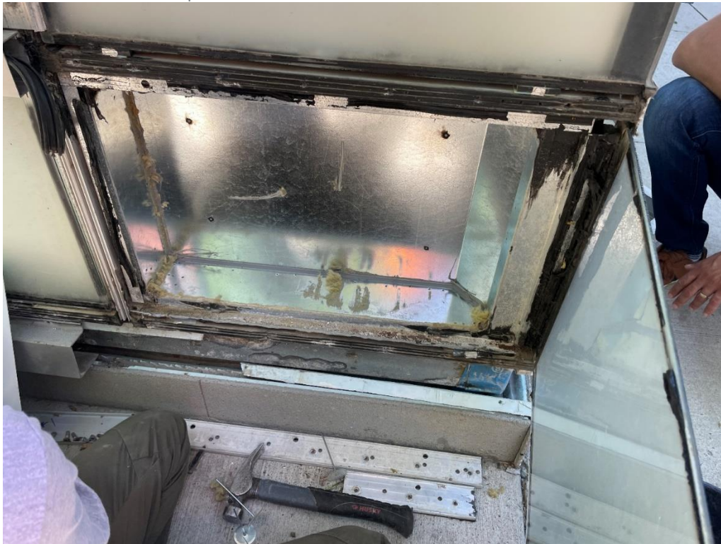
Photograph No. 36 Spandrel glazing and metal panel behind with removed insulation.
