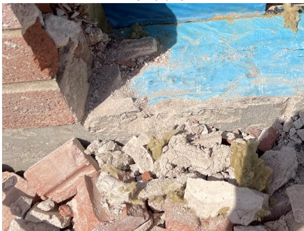
Image 15 – Mortar bed and parging
