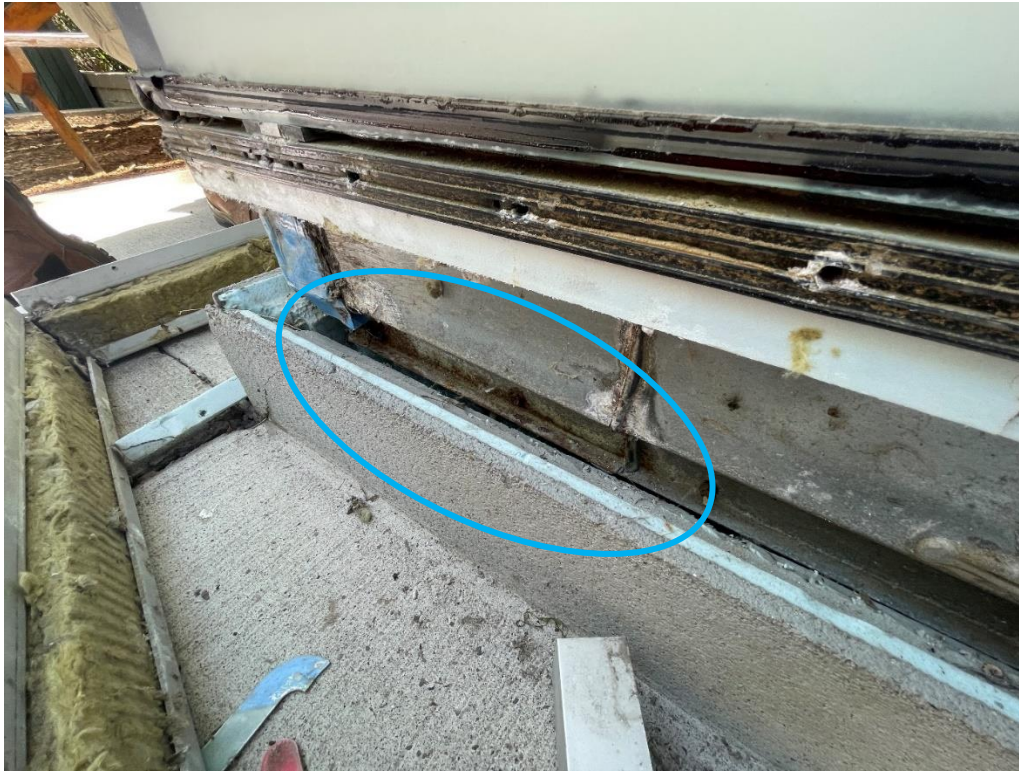
Photograph No. 35 Corroded metal closure panel on east elevation
