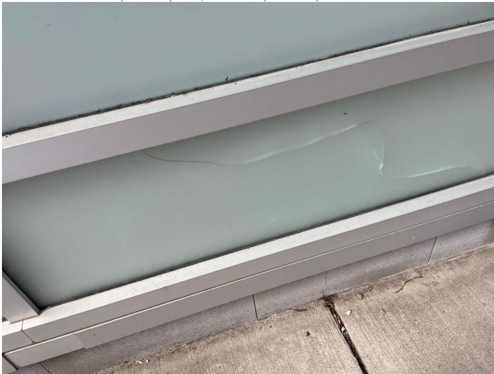
Photograph No. 16 Cracked spandrel glass.
