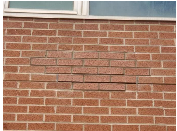
Image 28 – Example test opening re-instated
