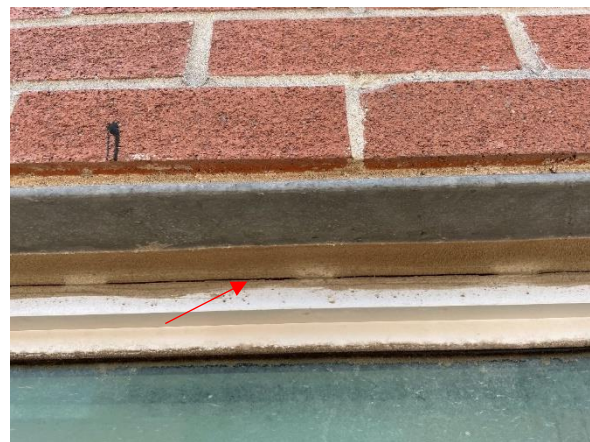
Image 8 – Debonding sealant
