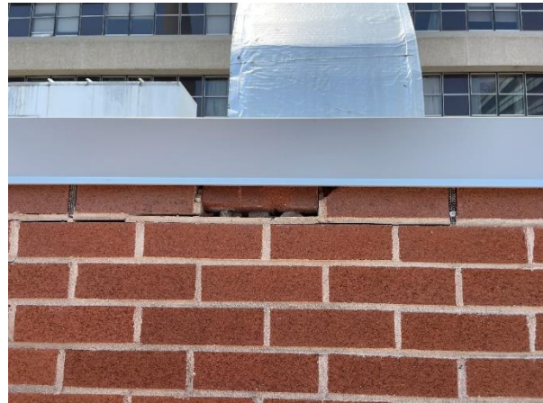
Image 6 – Loose bricks / cracking mortar
