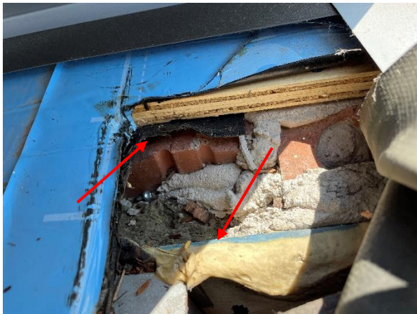
Image 25 – Wall WRB tie-in to mod. bit. membrane
