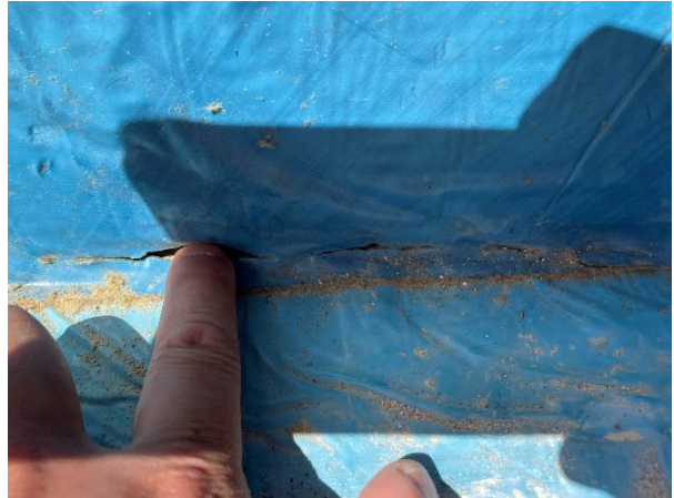
Image 12 – Hole in membrane
