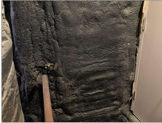
Photo 1 - Black coating on sprayed insulation, 19 th Floor
