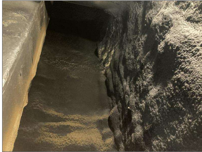
Photo 3 - Black coating on sprayed insulation, 6 th Floor
