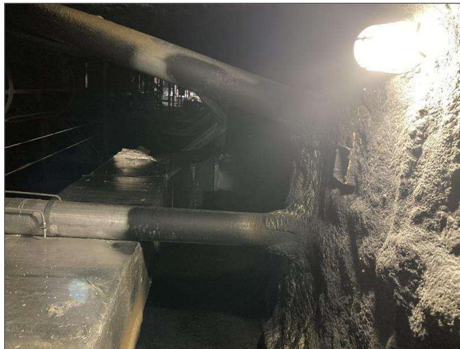
Photo 2 - Black coating on sprayed insulation, 12 th Floor
