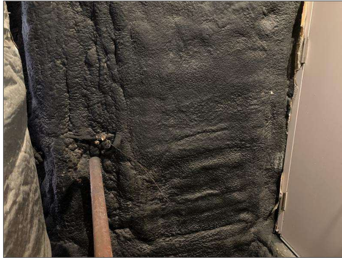
Photo 1 - Black coating on sprayed insulation, 19 th Floor
