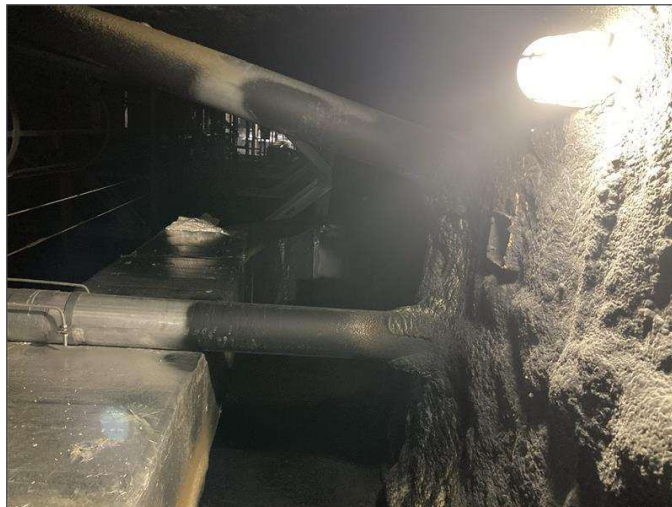
Photo 2 - Black coating on sprayed insulation, 12 th Floor
