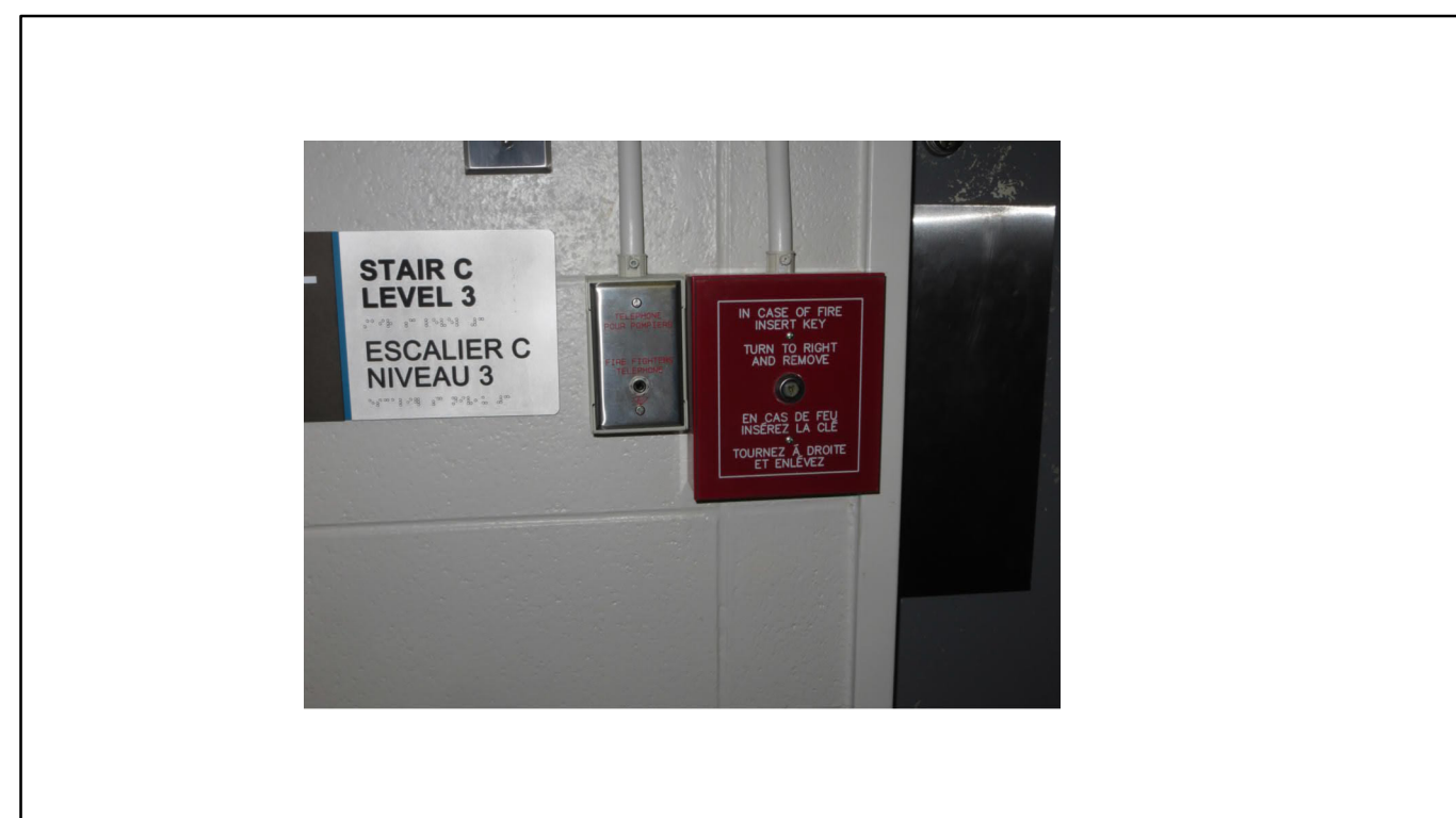
7 PHOTO OF EXISTING KEY SWITCH/MAN PULL STATION
