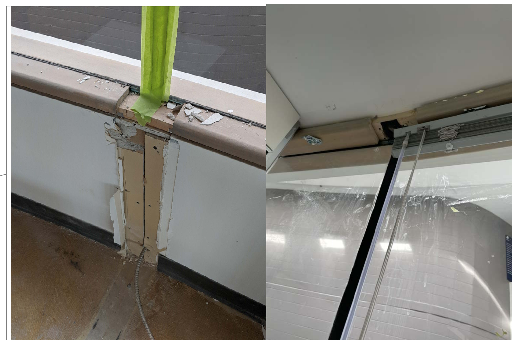
TYPICAL SITE CONDITION AFTER REMOVAL OF WALL FIN. REFER TO KEYNOTE #1
