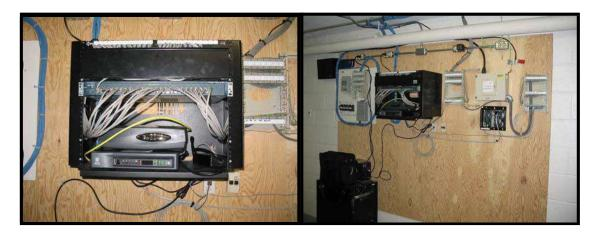
The HDSL circuit installed in this rack at the Fire Hall, 280 Burnhamthorpe. This is a little smaller than above. Only issue Patch cords should have been smaller, 2ft to hide in the cable manager. Almost 22 Connections. This room has enough space for a 2-post rack if required.
