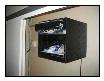
Currently the HDSL was not moved over from other location. This is the High Park supervisor's house. Issue here, rack was larger than expected by the client, so it should have been placed in the basement out of the way. That is why the closet now has doors. Rack is 11U Rack. There is about 12 connections in Total.
