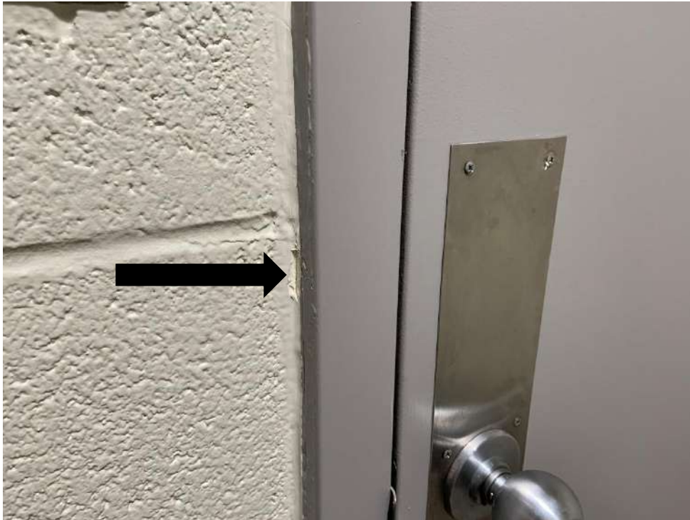
Photo 1 – View of the asbestos-containing cream caulking along the joint of a brick wall and a door frame.
