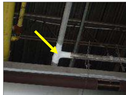
Photo 4: Repaired asbestos-containing parging cement on a tee in the Garage.
