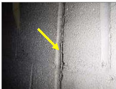
Photo 9: Asbestos-containing white caulking in Location 1-34 Garage.
