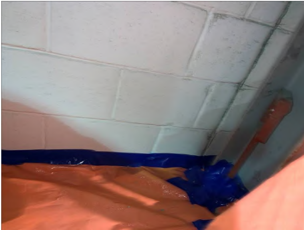
Photo 1: Example of the work area preparation for Type 1 removal.
