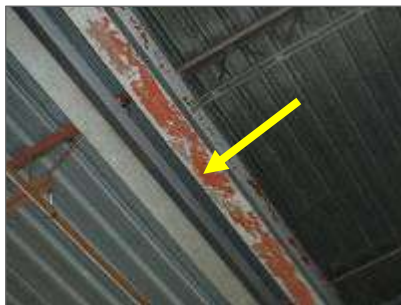
Photo 14: Flaking/peeling grey/red paint on structural beams in the Garage.
