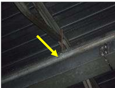
Photo 3: Asbestos-containing parging cement on a hanger in the Garage.
