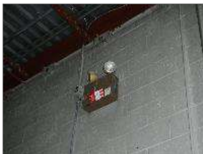
Photo 15: Emergency lighting in the Garage.
