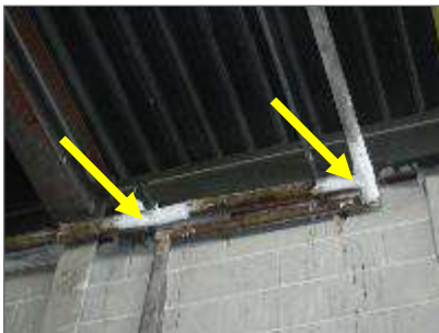
Photo 5: Repaired asbestos-containing parging cement fittings in the Garage.
