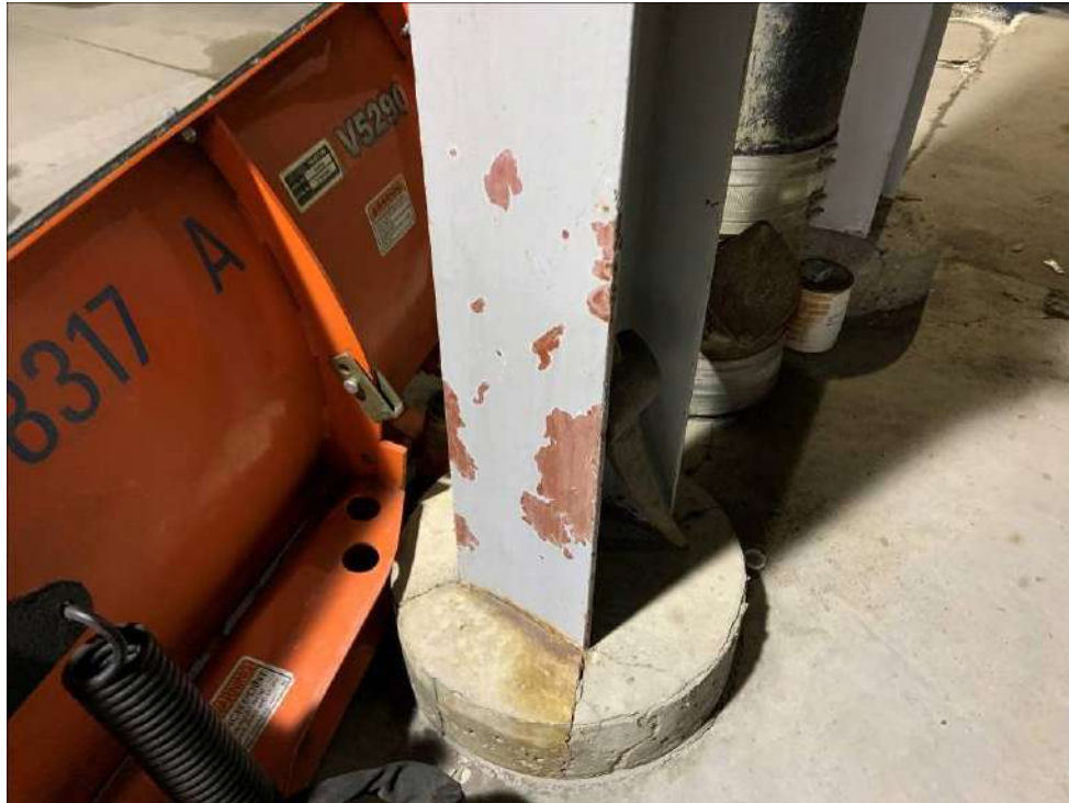
Photo 15: Post abatement view of a metal column after removal of the lead-containing flaking and loose paint.
