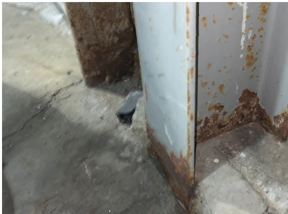
Photo 16: Another post abatement view of a metal column after removal of the lead-containing flaking and loose paint.
