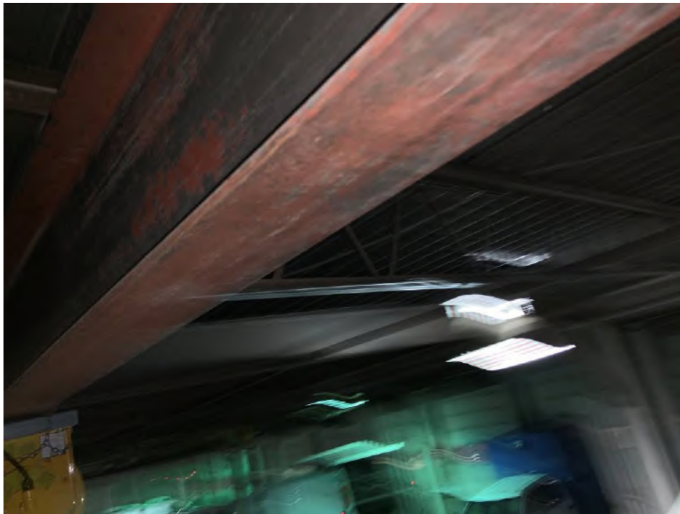
Photo 14: Another post abatement view of a metal beam after removal of the lead-containing flaking and loose paint.
