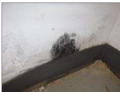
Photo 16: Visible mould growth on drywall in the 1-73 Vestibule.
