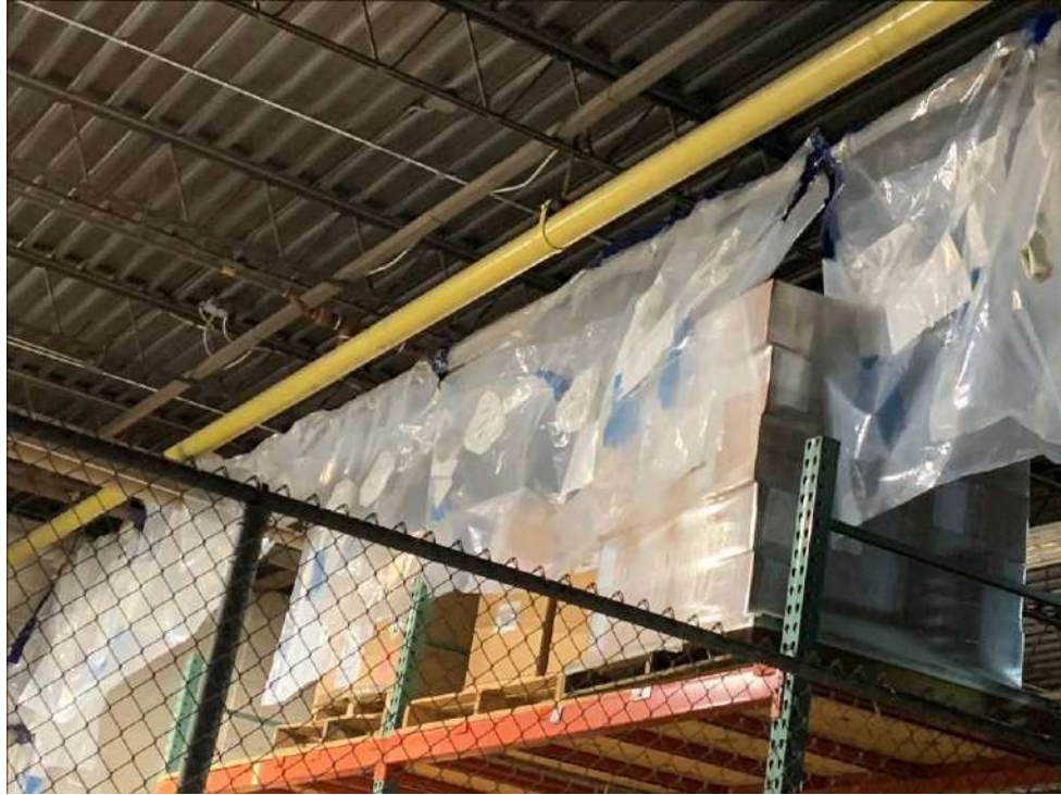
Photo 9: View of the Glove Bag settings for removal of the asbestos-containing air-cell on a pipe straight.
