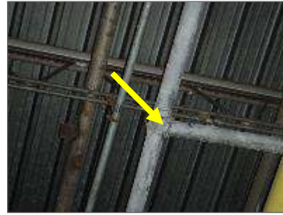
Photo 2: Asbestos-containing parging cement on a tee in the Garage.
