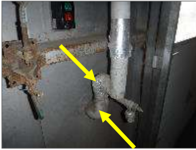
Photo 1: Asbestos-containing parging cement on an elbow in the Garage.
