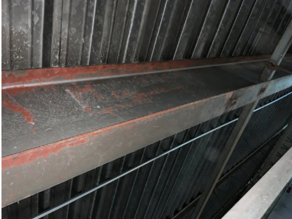
Photo 13: Example of the post abatement view of a metal beam after removal of the lead-containing flaking and loose paint.
