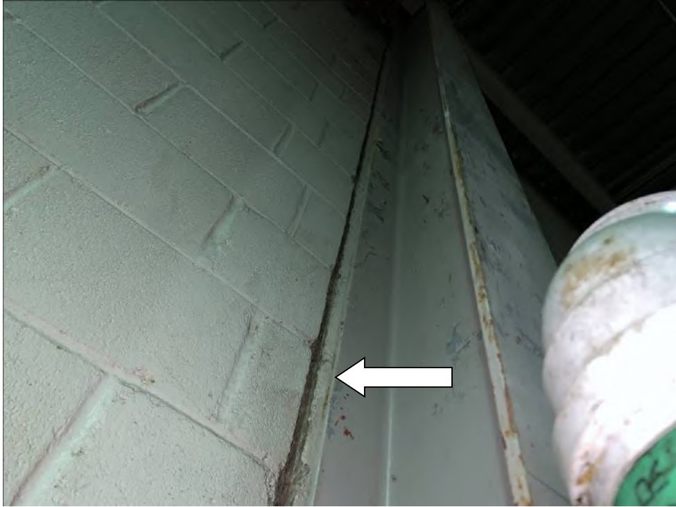
Photo 3: Example of the post abatement view of the wall joint behind the metal column.
