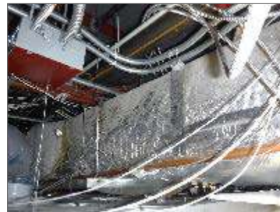
Photo 6: Duct insulated with fibreglass and jacketed in foil present in Corridor (Location 2-140).
