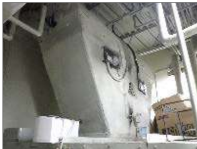
Photo 5: Duct insulated with fibreglass and jacketed in canvas present in Mechanical Room (Location 1-106).
