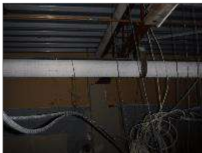
Photo 13: Transite pipe present above acoustic ceiling tile in Office (Location 2-088).
