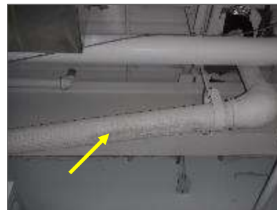
Photo 14: Transite pipe present Men's/Women's Change Room (Location 2-145).
