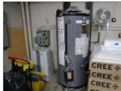
Photo 8: Hot water tank present in Boiler Room (Location B-014).
