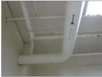
Photo 3: Hot water supply pipe insulated with fibreglass present in the Basement Document Storage room (Location B-013).
