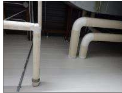
Photo 4: Pipes insulated fibreglass present in the Rooftop Mechanical Room (Location 4-001).
