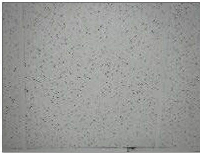
Photo 9: Assumed asbestos-containing ACT10.
