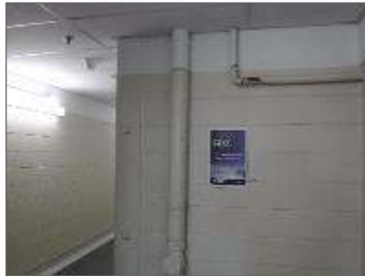
Photo 15: Transite pipe present in Corridor (Location 1-098).
