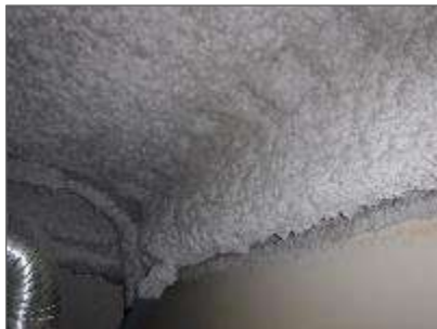
Photo 1: Non-asbestos fireproofing present above acoustic ceiling tile in the Automotive Parts room (Location 1-032).
