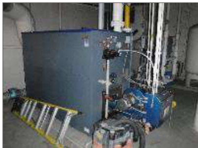
Photo 7: Boiler present in Boiler Room (Location B-014).
