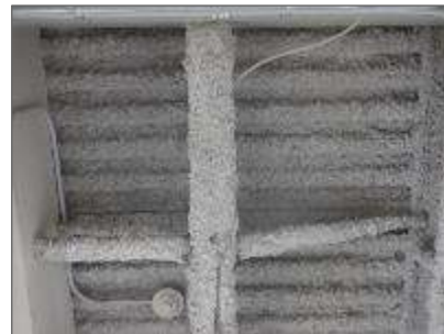
Photo 2: Non-asbestos fireproofing present in Elevator Mechanical Room (Location 1-050).
