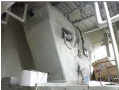
Photo 5: Duct insulated with fibreglass and jacketed in canvas present in Mechanical Room (Location 1-106).
