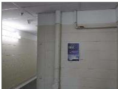
Photo 15: Transite pipe present in Corridor (Location 1-098).
