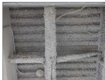
Photo 2: Non-asbestos fireproofing present in Elevator Mechanical Room (Location 1-050).
