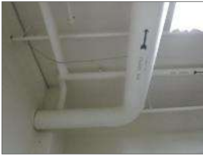
Photo 3: Hot water supply pipe insulated with fibreglass present in the Basement Document Storage room (Location B-013).
