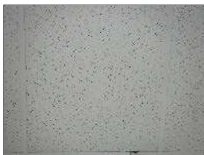
Photo 9: Assumed asbestos-containing ACT10.
