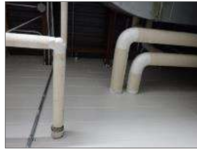
Photo 4: Pipes insulated fibreglass present in the Rooftop Mechanical Room (Location 4-001).
