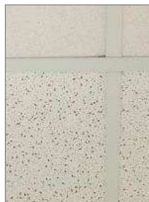
Photo 4: Non-asbestos ACT03 in the Office (Location 1-05).
