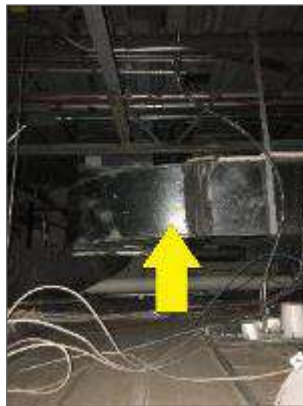
Photo 2: Uninsulated duct above the ceiling tiles in the Office Area (Location 1-04).
