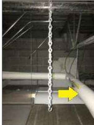
Photo 1: Pipe insulated with fibreglass above the ceiling tiles in the Corridor (Location 1-02).
