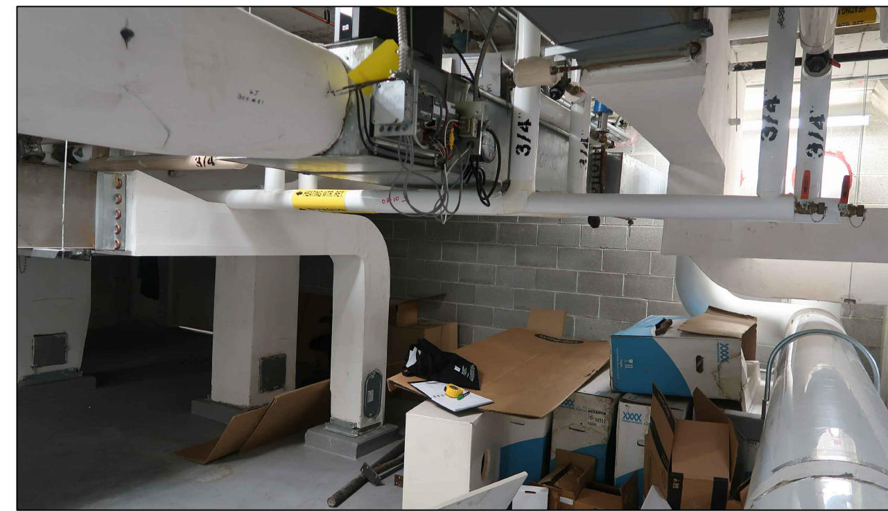
LOCATION OF NEW DUCT PENETRATION REQUIRED LOOKING EAST 6 A00-05
