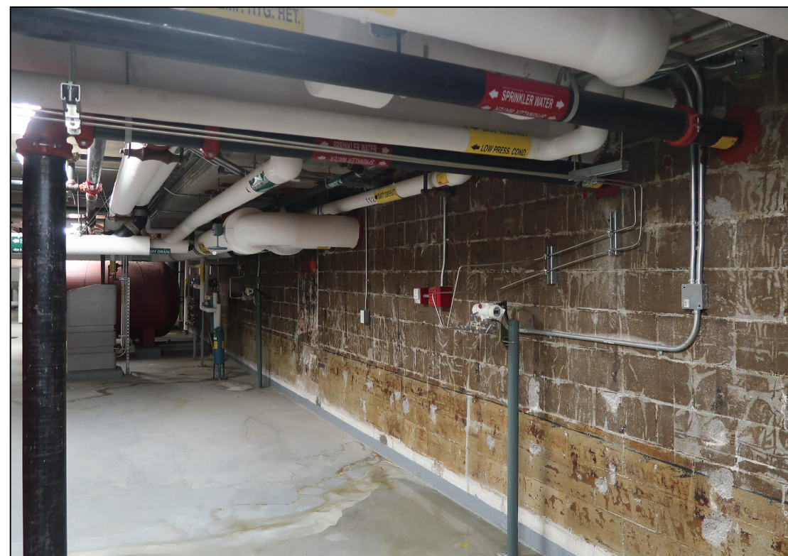
EXIST SERVICES IN MECH ROOM M3-700 LOOKING S-W 12 A00-05
