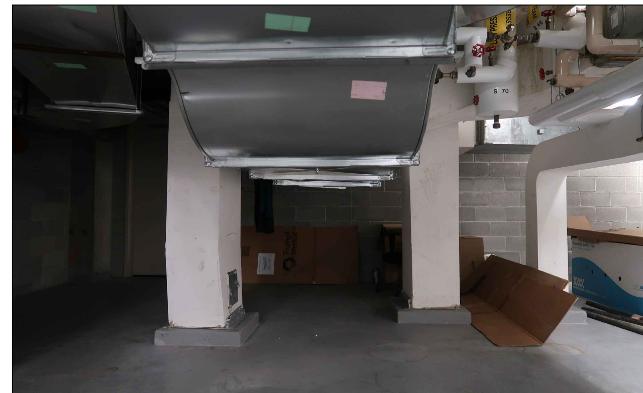
EXISTING DUCT SERVICES AT MECHANICAL ROOM EAST WALL 8 A00-05
