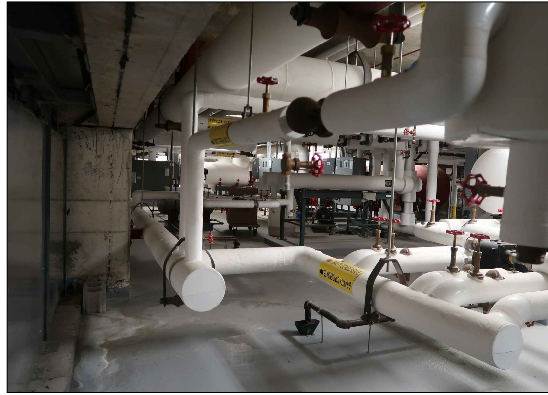
MECHANICAL ROOM M3-700 LOOKING SOUTH 15 A00-05
