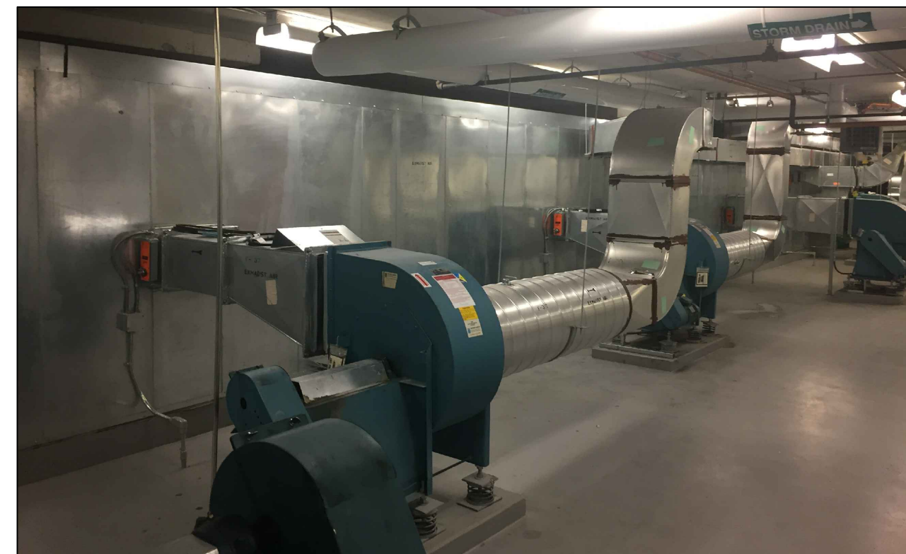
MECHANICAL ROOM AREA LOOKING NORTH-EAST 4 A00-05
