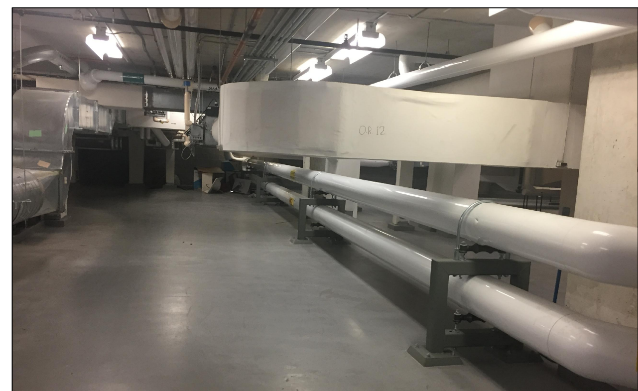
MECHANICAL ROOM AREA LOOKING EAST 5 A00-05
