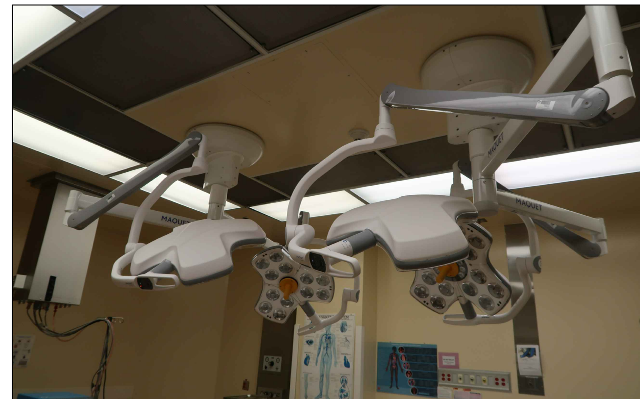
OR SUITE #14 VIEW OF EXISTING CEILING (8) A00-04
