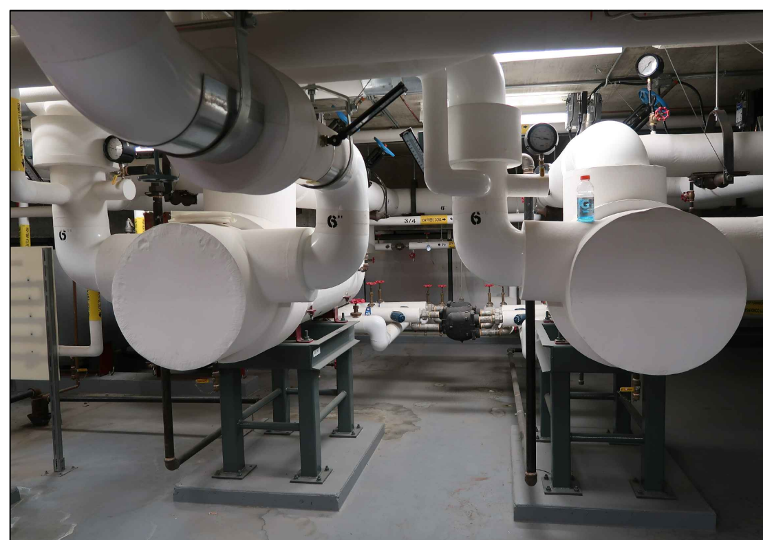
MECHANICAL ROOM M3-700 LOOKING EAST 13 A00-05
