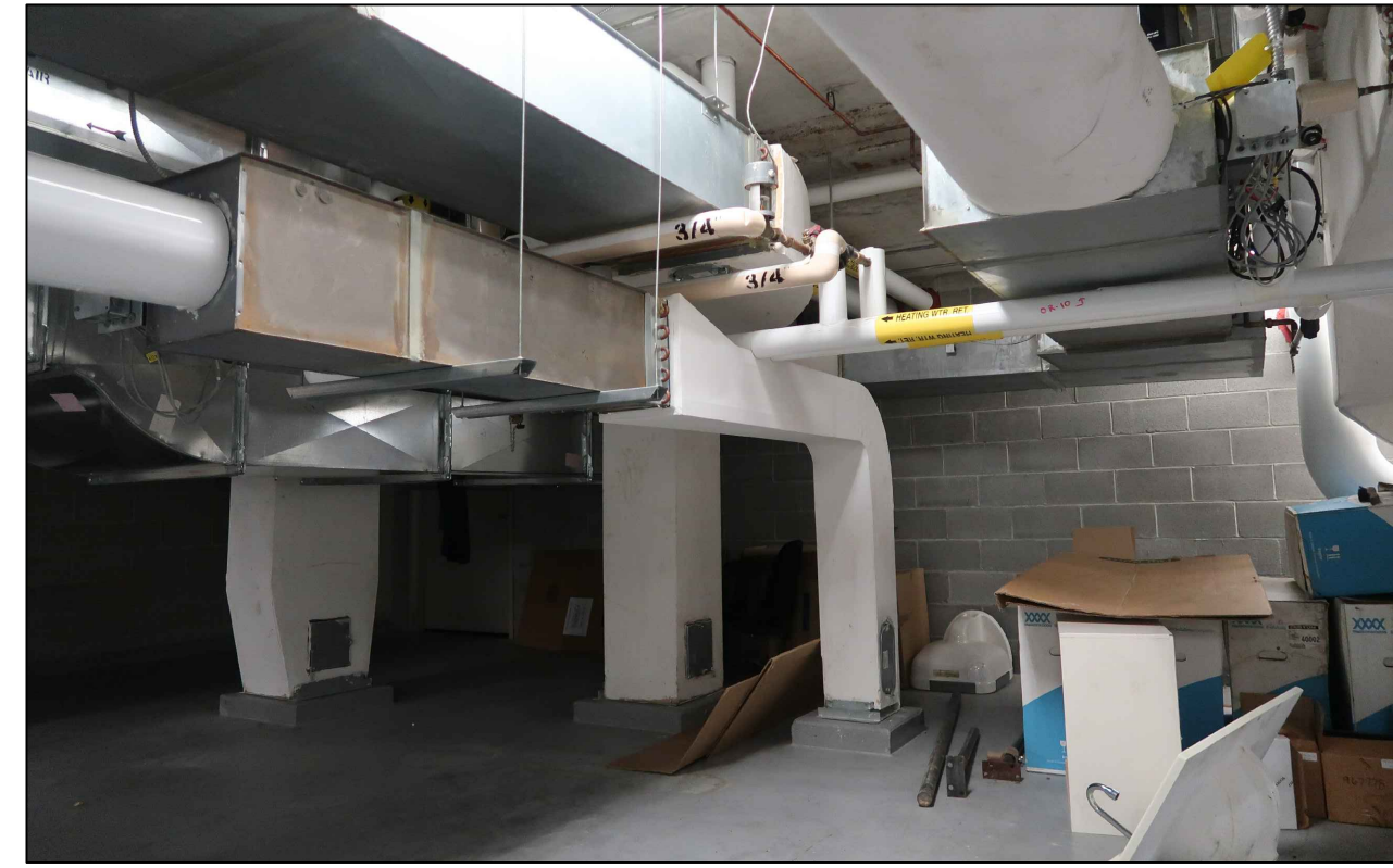
EXISTING DUCT SERVICES AT MECHANICAL ROOM EAST WALL 7 A00-05
