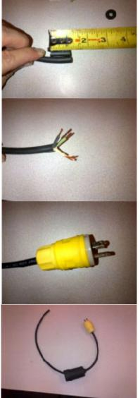
1. Remove 1" of cab tire casing & strip wires at each end
