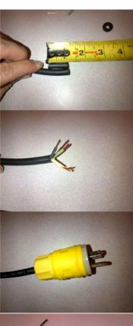
1. Remove 1" of cab tire casing & strip wires at each end
