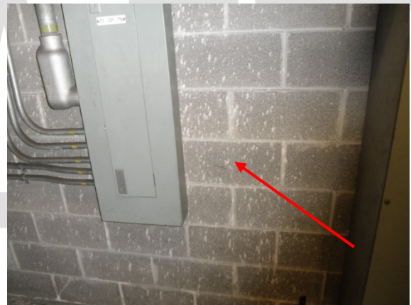
4 – View of non-asbestos overspray material in Room 51P-304 (Concourse Level).
