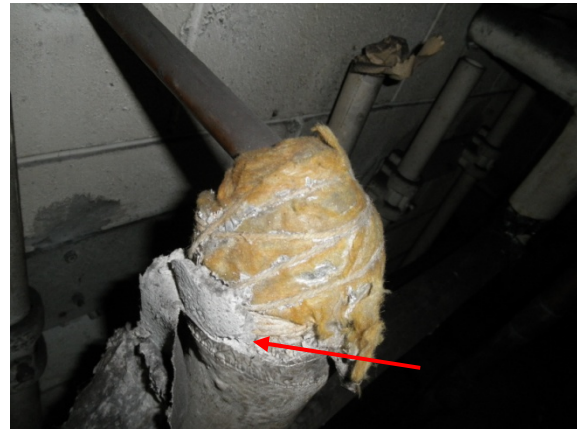
2 – View of non-asbestos parging cement on pipe fittings in Room 21Y-18 (Street Level).
