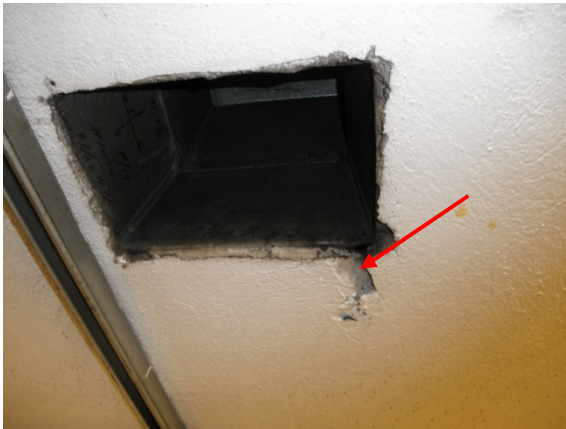
1 – View of asbestos-containing plaster in Room 21Y-68 (Platform Level).
