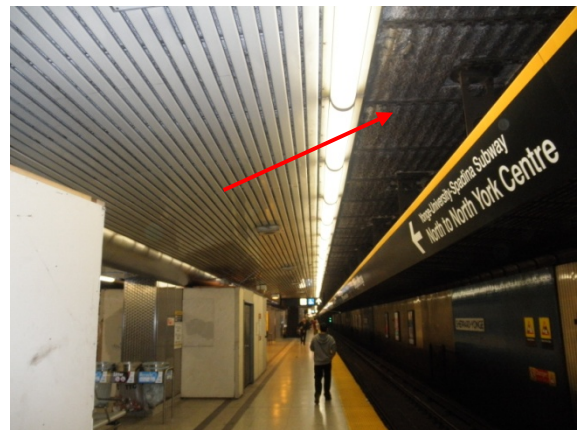
6 – View of asbestos-containing spray on fire proofing the deck (Track Level).
