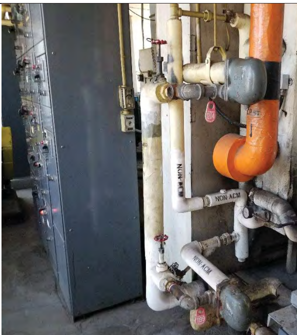
Photo 19: Parged wrapping remediation efforts observed in Penthouse 222.
