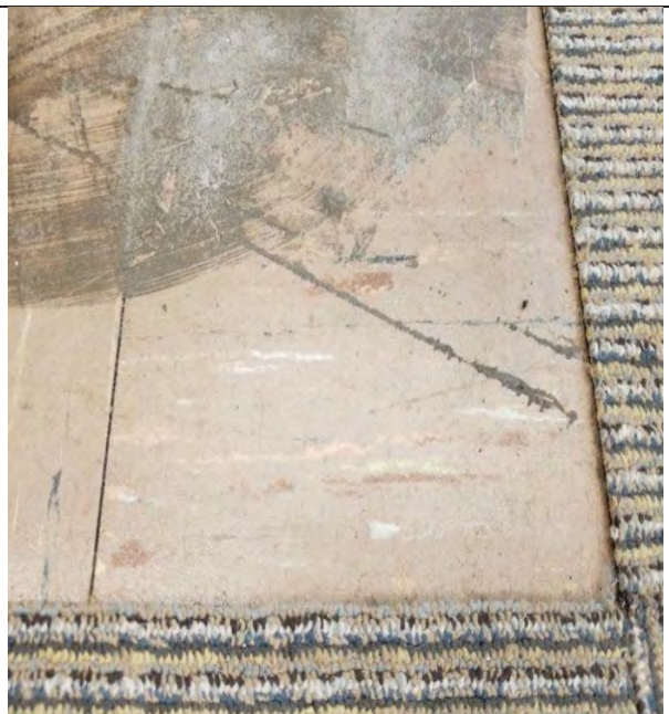
Photo 8: VFT – Brown with multi-colour streaks 9x9 (LEX sample 30). 0.5% Chrysotile.
