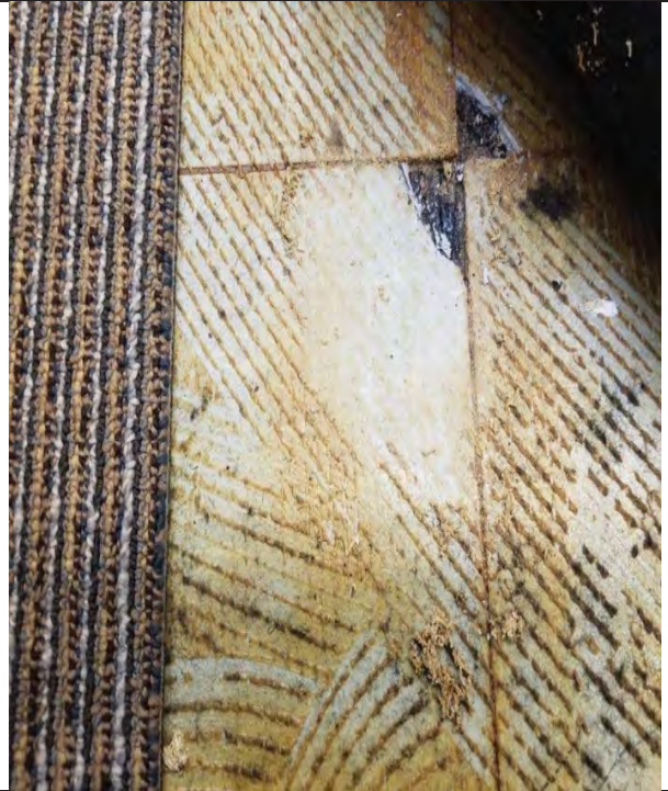
Photo 14: VFT – Grey with white 9x9 (LEX sample 18). 0.5% Chrysotile.
