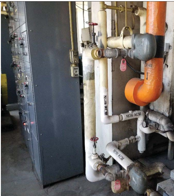
Photo 19: Parged wrapping remediation efforts observed in Penthouse 222.
