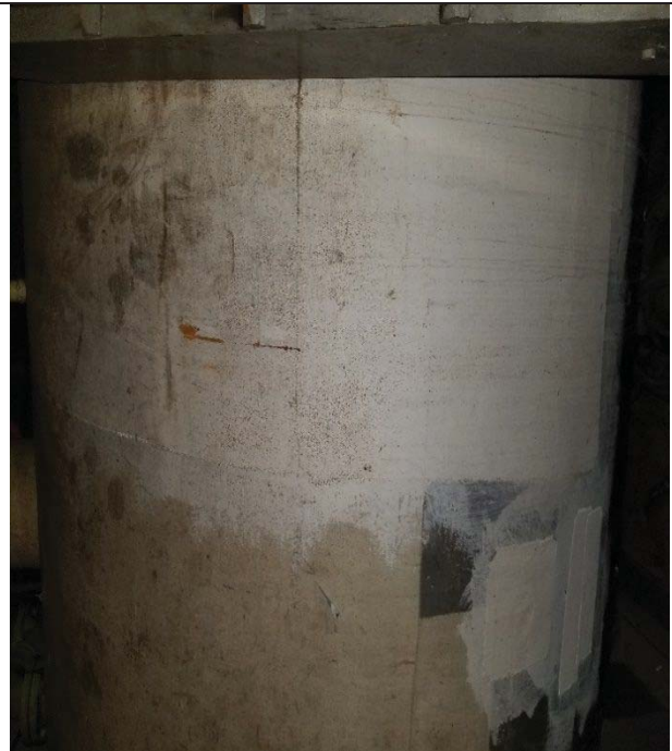
Photo 2: Parged pipe wrapping located in the Sewage Room 120A. Presumed asbestos containing.
