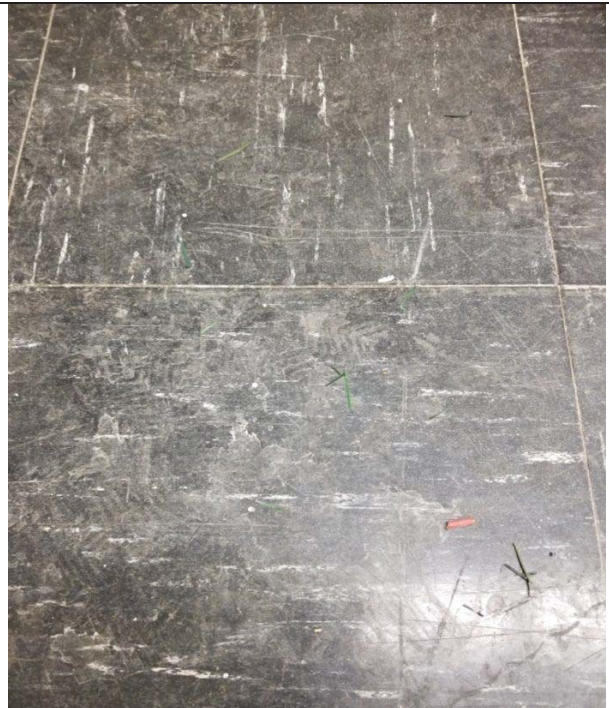
Photo 16: VFT – Black with white streaks (LEX sample 33). 6% Chrysotile
