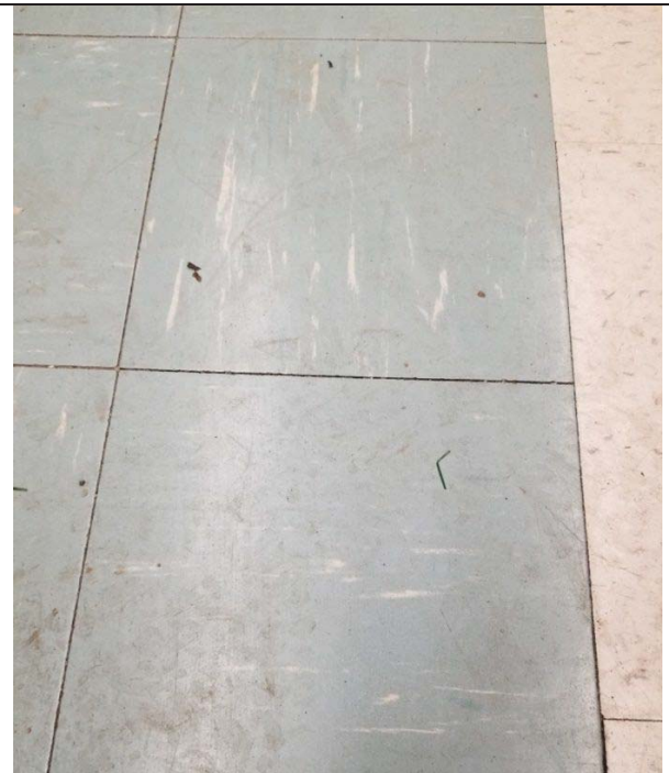
Photo 10: VFT – Blue with white streaks 9x9 (LEX sample 32). 1% Chrysotile.
