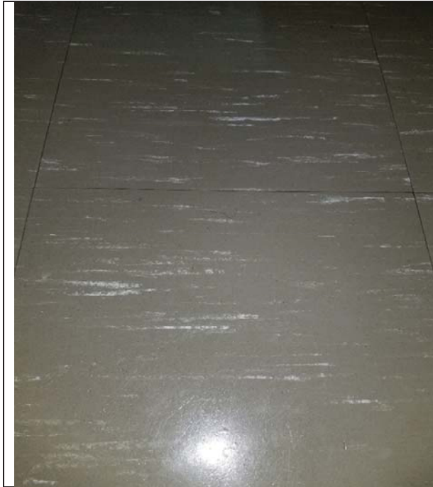
Photo 17: VFT – Army green with white (LEX sample 39). 1% Chrysotile.
