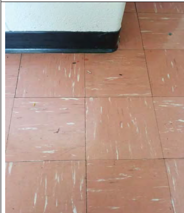
Photo 11: VFT – Red with white streaks 9x9 (LEX sample 36). 1% Chrysotile.
