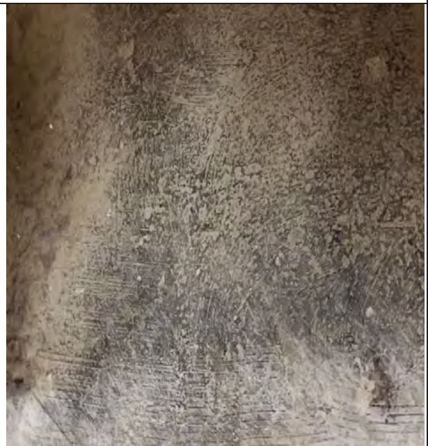
Photo 4: Black VFT mastic found throughout the building. 1% Chrysotile.
