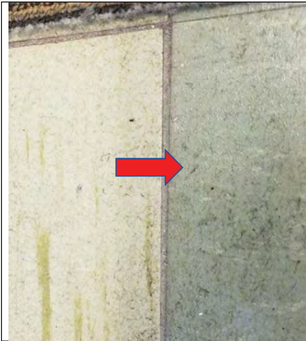
Photo 5: VFT – Teal with white streaks (Right tile, LEX sample 23). 1% Chrysotile.
