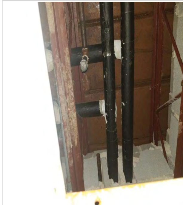
Photo 1: Parged pipe fitting found throughout the building. 50% Chrysotile.
