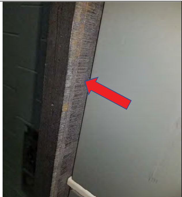
Photo 18: Transite bench board found in room 138. Presumed asbestos containing.
