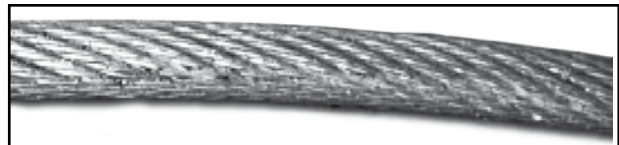
Outside of wire rope. It appears to be in good condition. See below.
